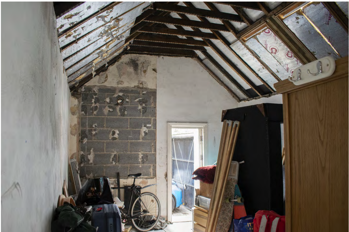
Plate 27 Rear extension with infilled window and skylights.
