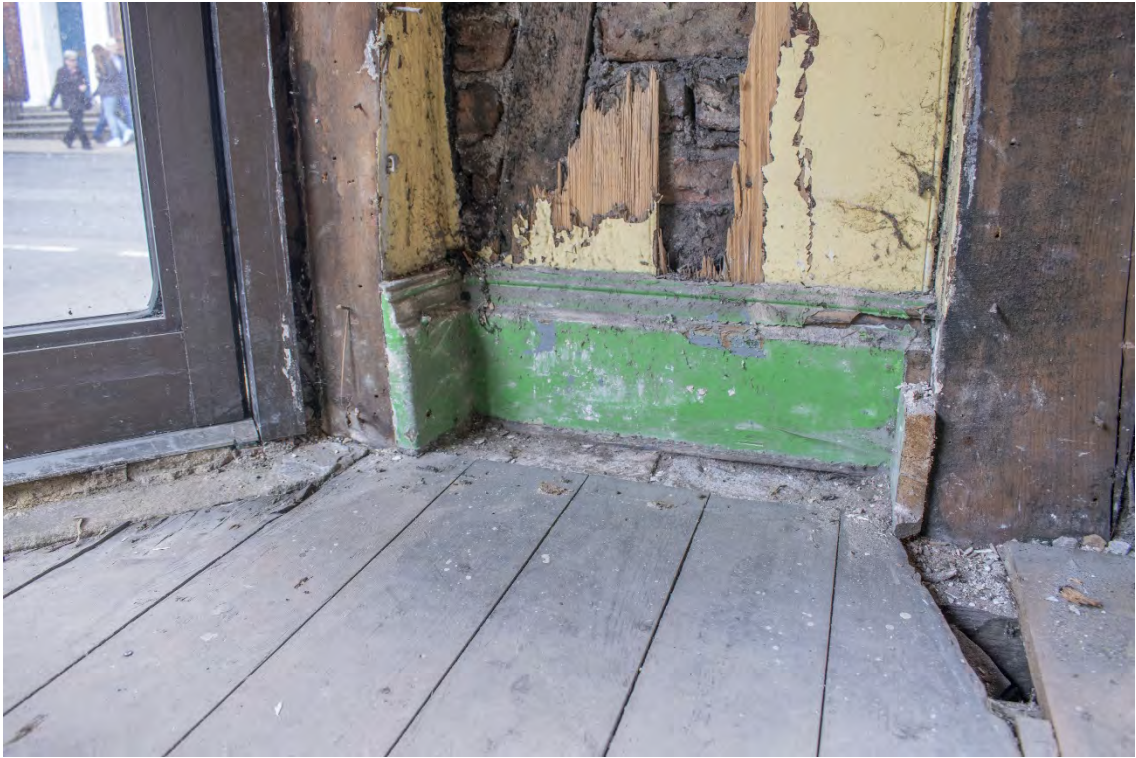
Plate 11 Original skirting detail.
