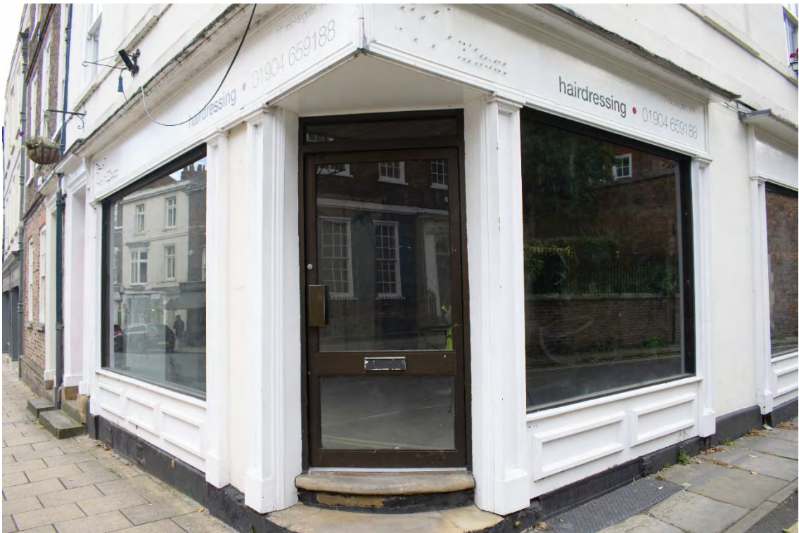
Plate 4 Canted corner door, mid-20th century addition.
