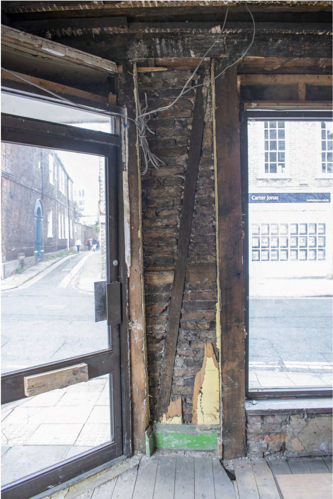
Plate 10 Recessed section of wall with exposed brick with timber brace. Original skirting detail.
