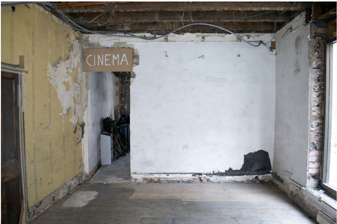
Plate 16 South wall with opening to rear extension.
