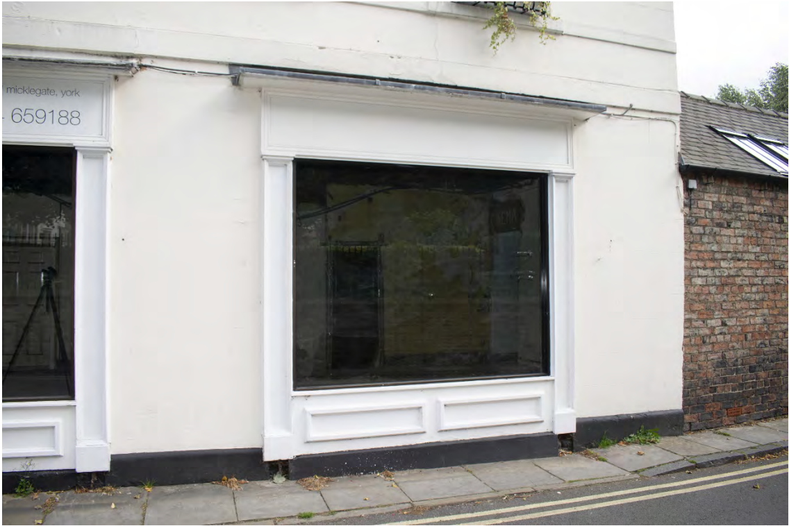
Plate 5 Example of shop frontage style on west facing elevation.
