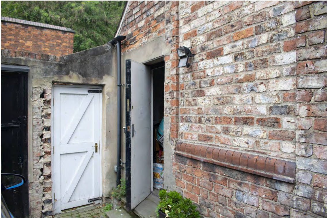
Plate 8 Rear door and infilled window with decorative brick sill.
