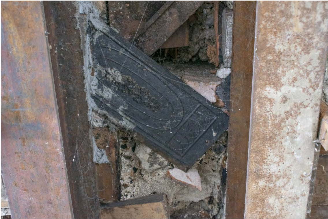
Plate 24 Metal fireback plate within rubble between steel beams.
