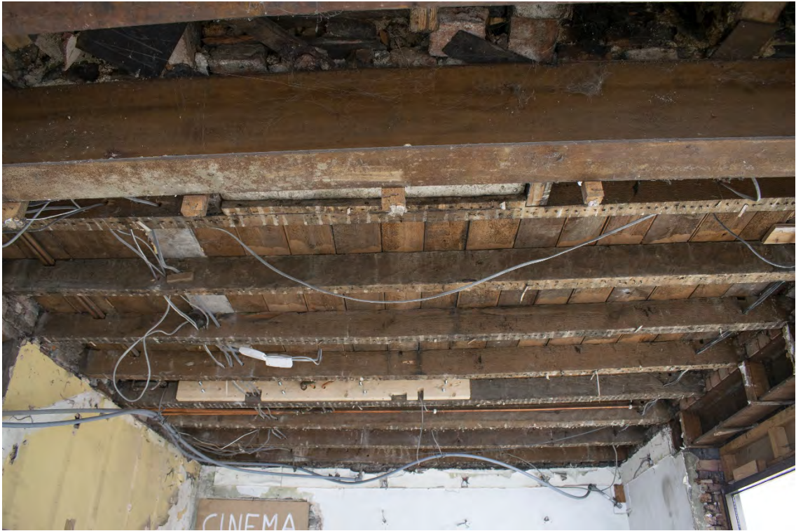
Plate 21 Rear ceiling and floor structure.
