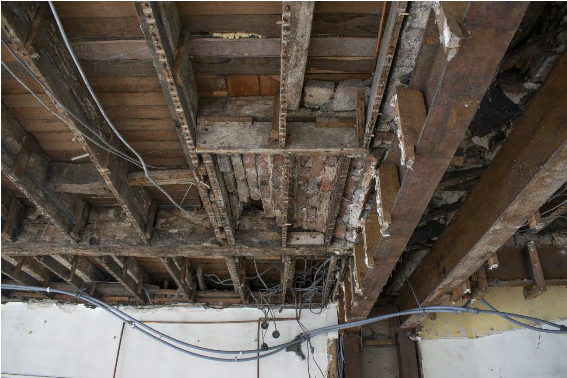
Plate 26 Brick chimney hearth with timber supports.
