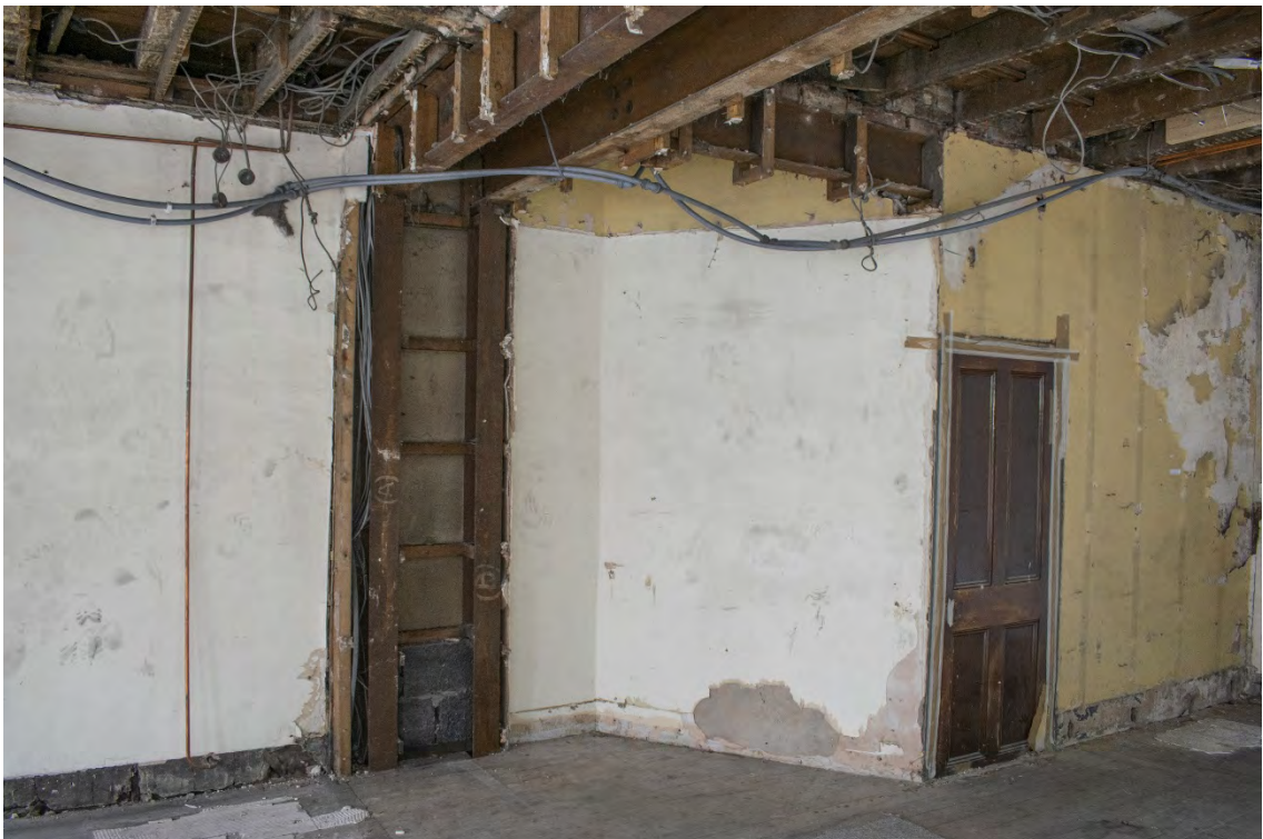
Plate 12 East wall with steel beams and re-opened interior doorway.
