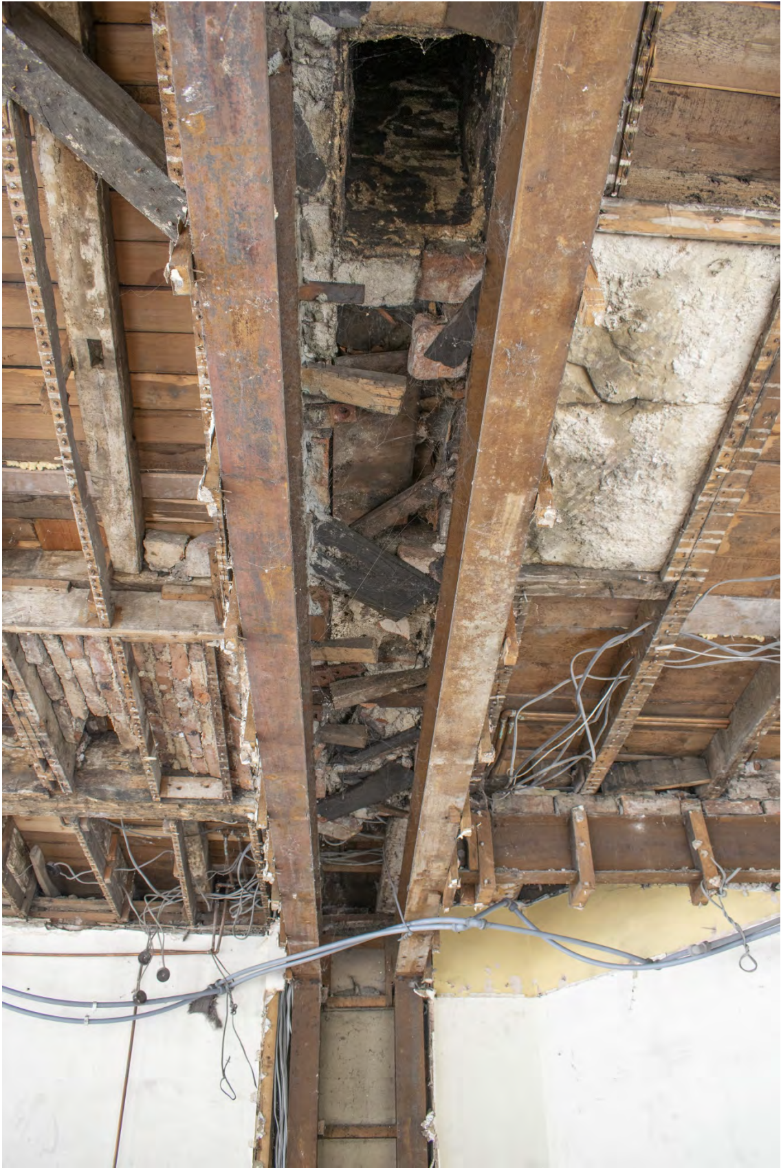
Plate 23 Chimney stone hearth and flue.
