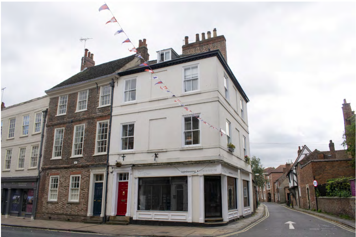
Plate 2 North facing elevation fronting onto Micklegate.
