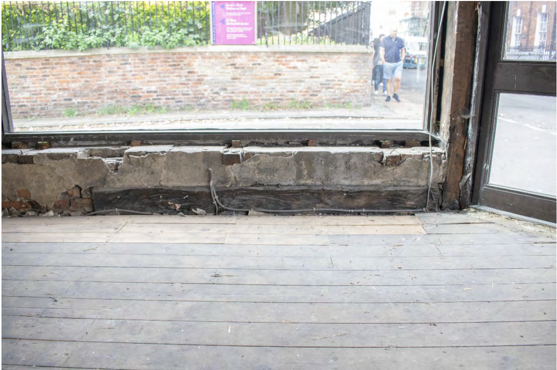
Plate 19 Original timber threshold beneath display window.
