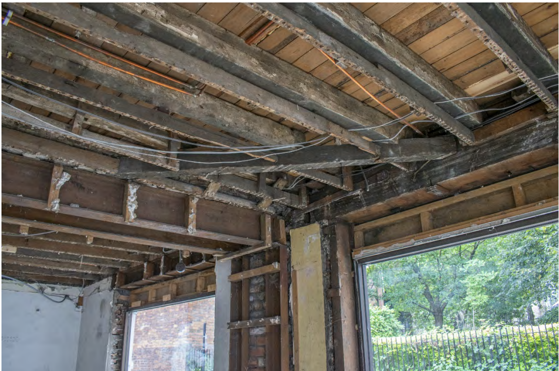
Plate 25 Diagonal support beam for chimney flue.
