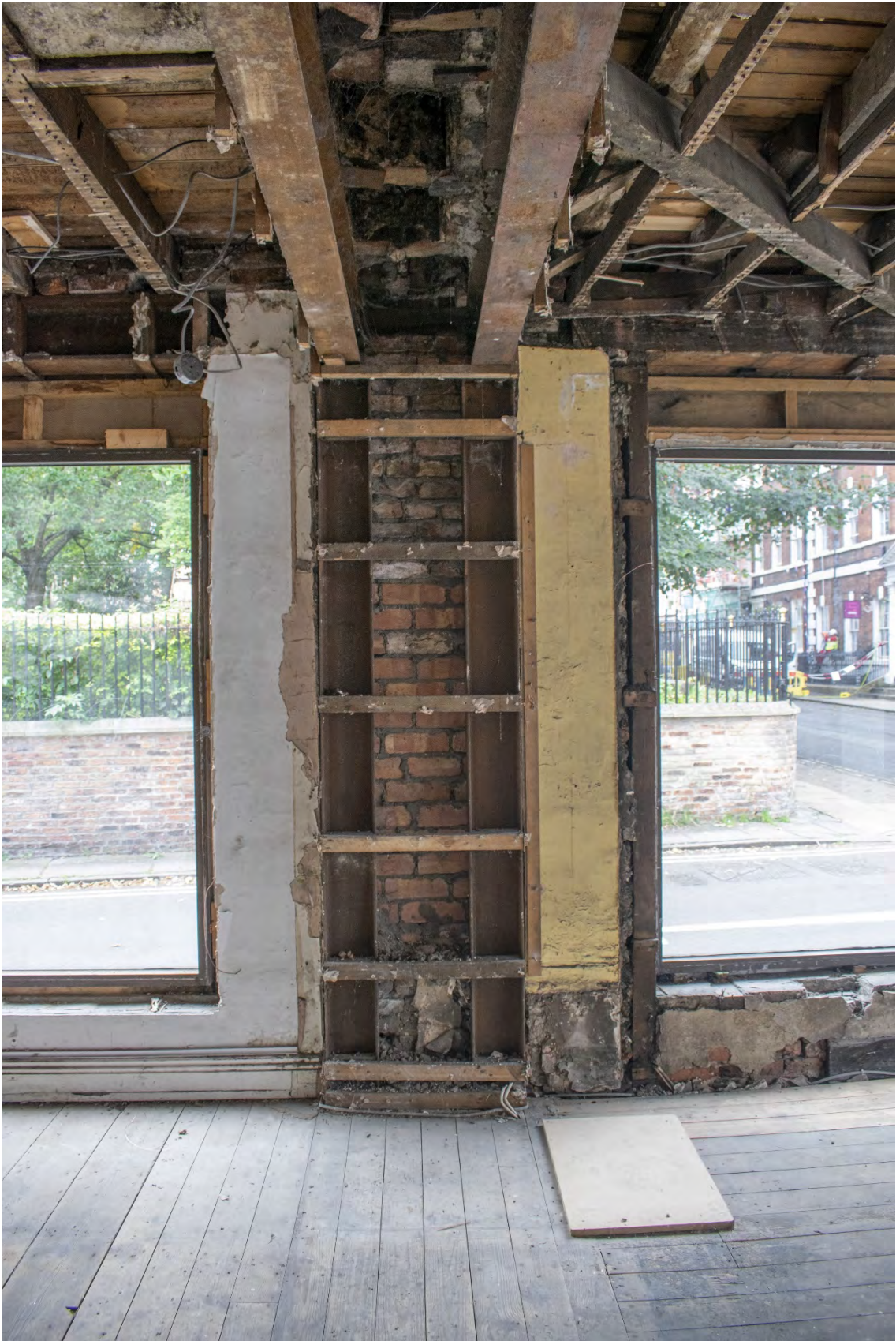
Plate 14 Structural steel beams replacing original dividing wall.
