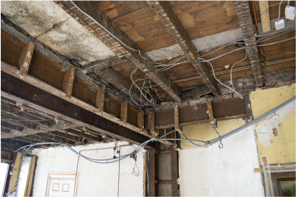
Plate 15 Structural steel beams aligned east/west and north/south.
