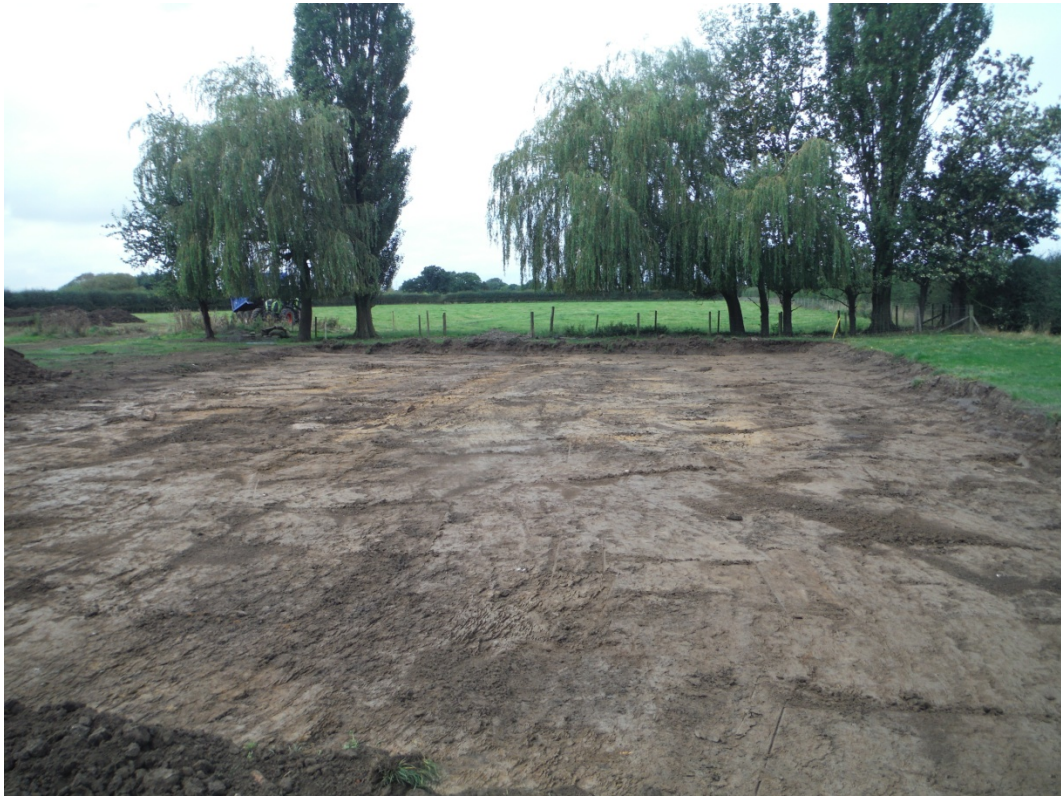
Plate 8 General area shot looking South West showing final stripped area.
