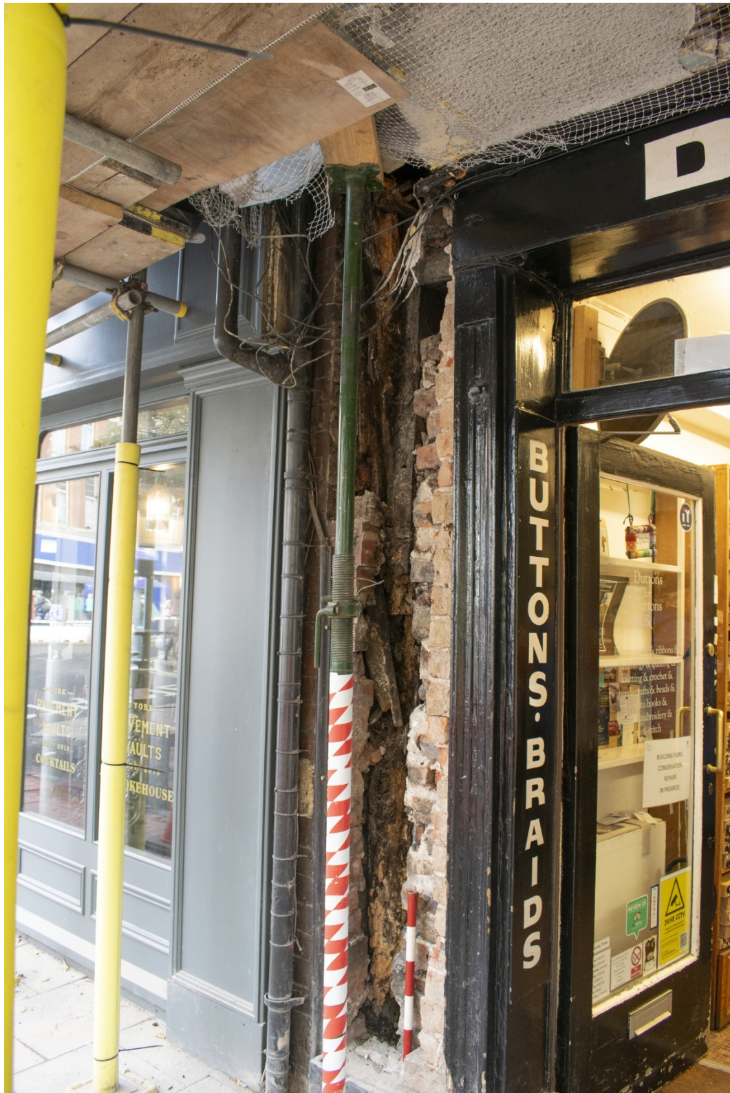
Plate 3 Ground Floor timber post on stone post pad.
