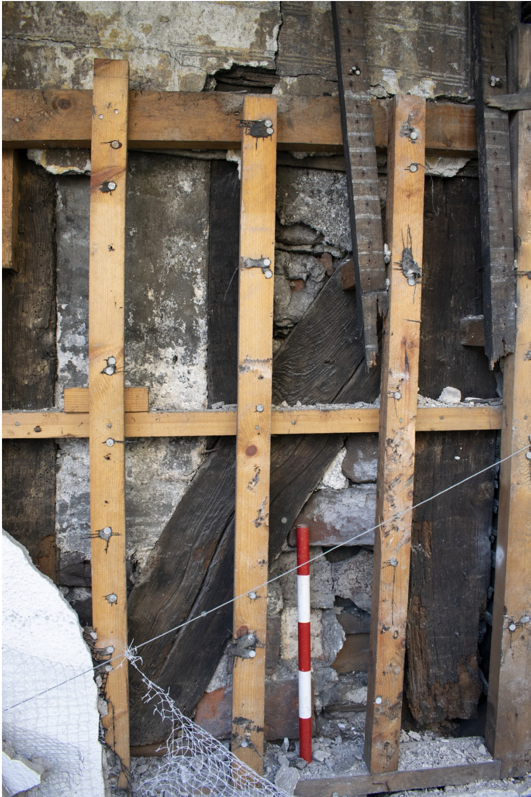
Plate 6 Detail of surviving timber frame on right side of jetty.
