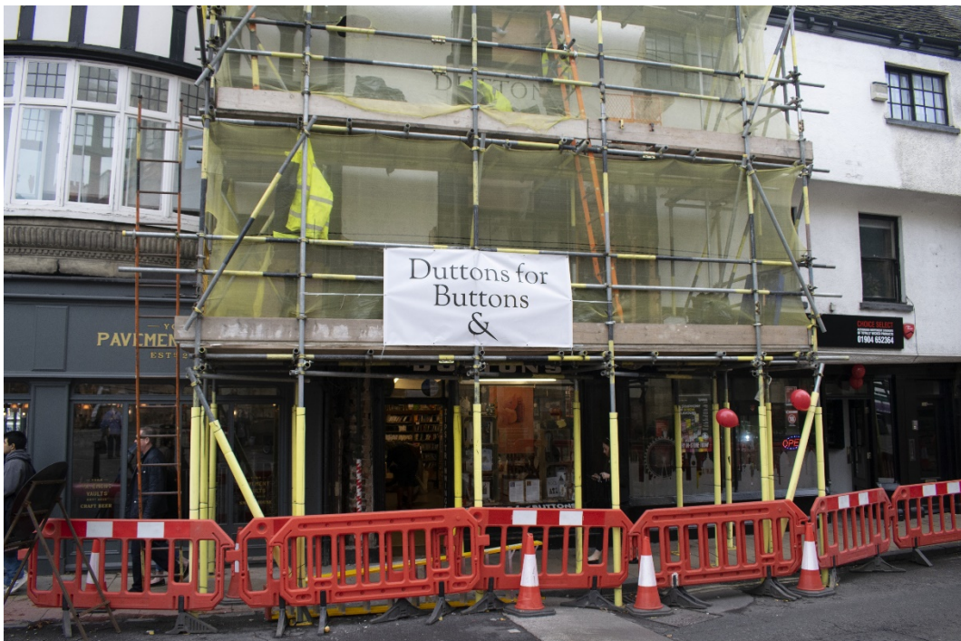
Plate 2 North-east facing elevation.
