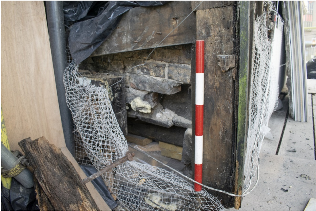
Plate 9 Floor structure with planks and timber beam.
