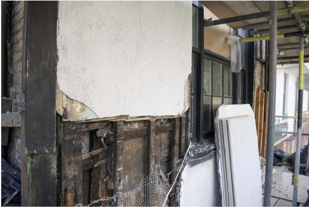
Plate 5 Overview of first-floor jetty works.
