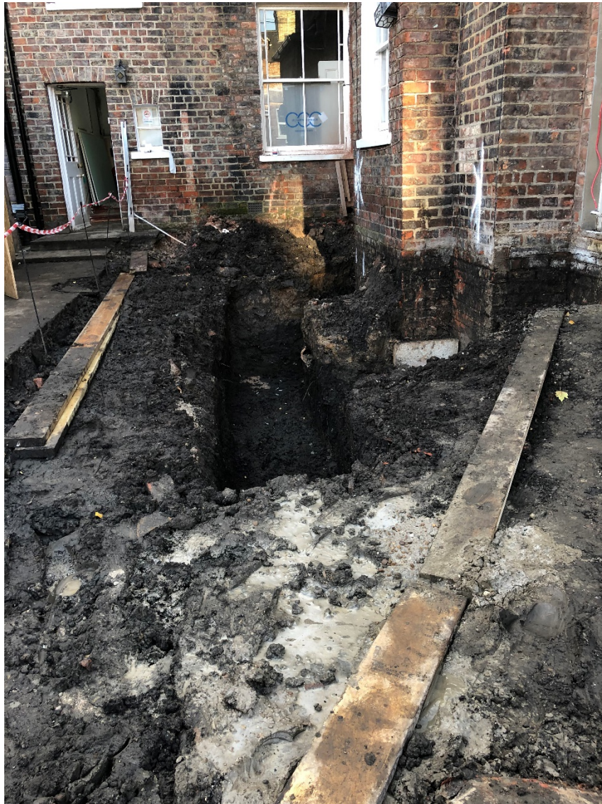
Plate 2 General site shot of the works, view south-west.
