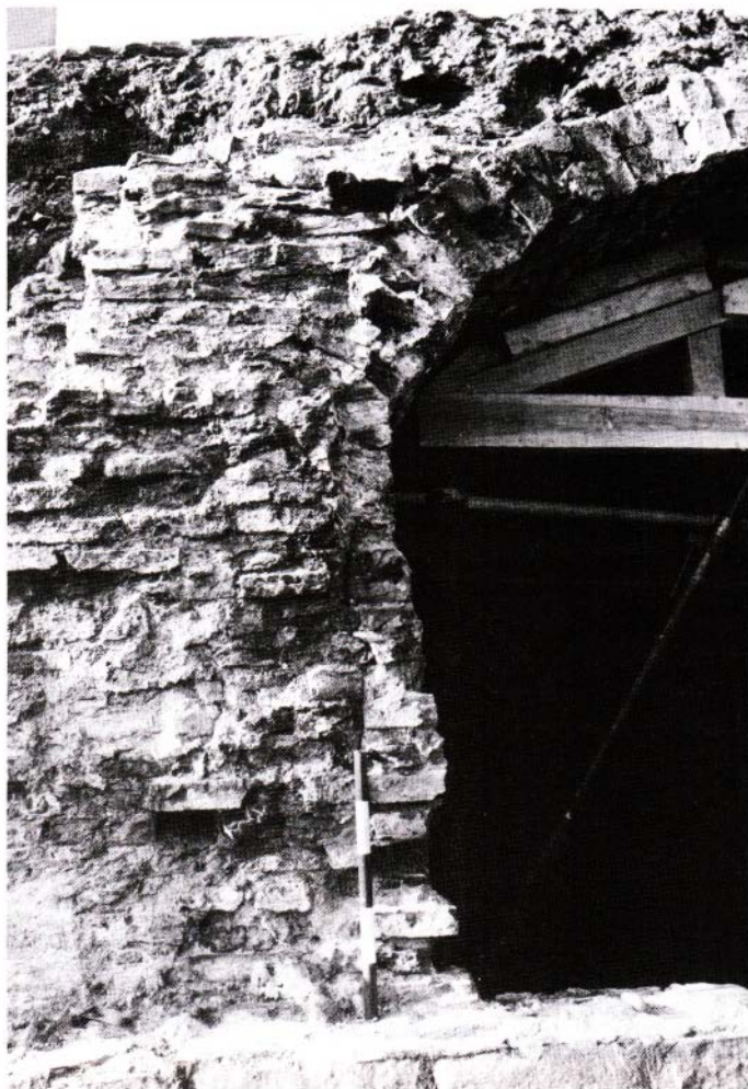
Tower 13: tower structure - limestone facing, brick vault, earth fill.
