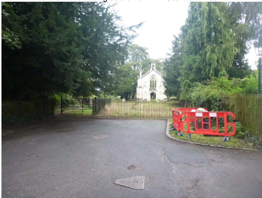
Plate 4 Working shot of Trial Pit 1
