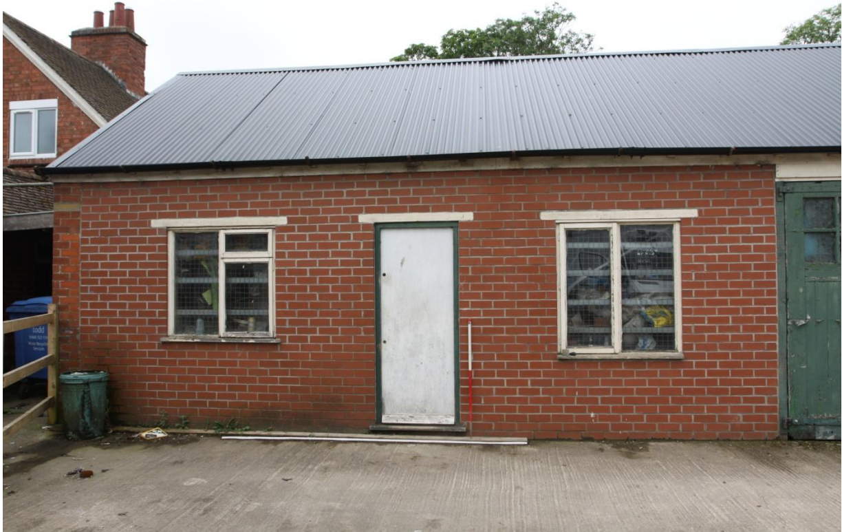
Plate 9 The north-eastern elevation of Unit A, view south-west.
