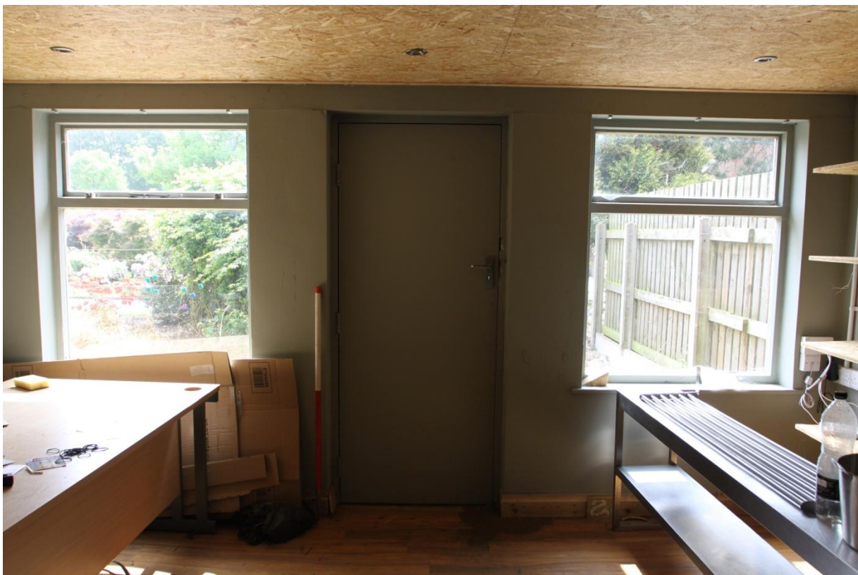
Plate 17 Later 20 th century extension on Unit B, view south-east.
