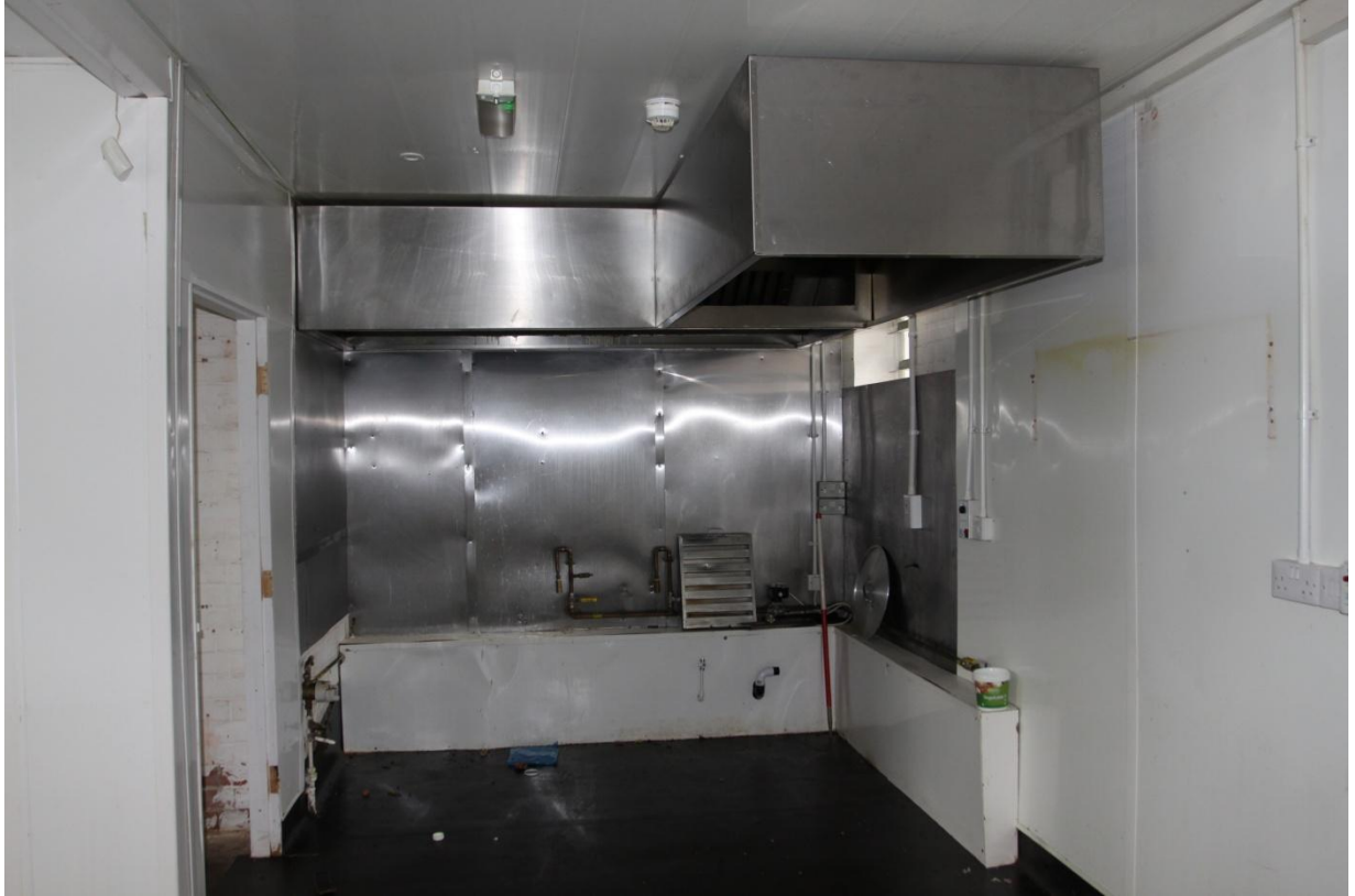
Plate 25 Kitchen in the main room of Unit D, view south-west.
