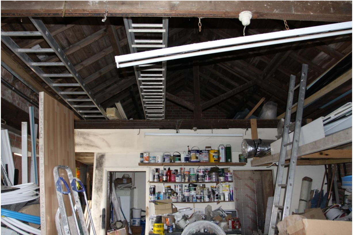
Plate 11 The interior of Unit A, view south-east.
