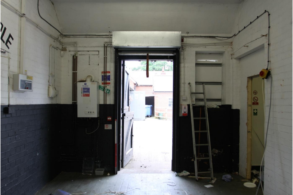
Plate 23 The stable door in the south-western wall of the central room in Unit D, view south-west.
