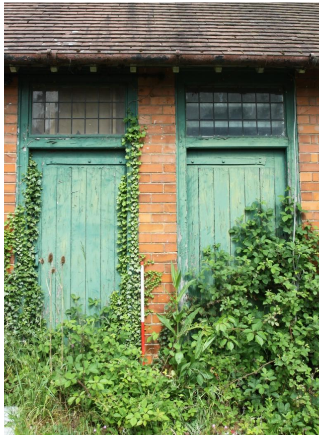
Plate 6 External view of the two doorways in Unit D, view north-west.
