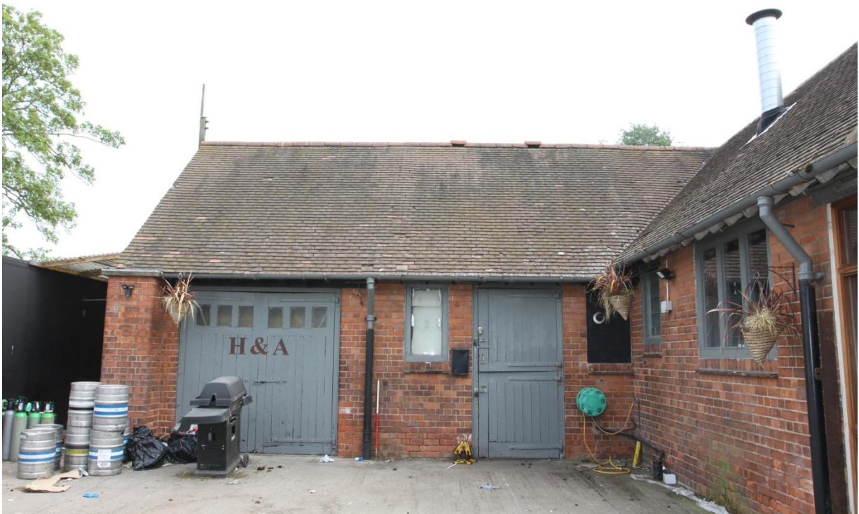
Plate 7 View of the south-western elevation of Unit D, view north-east.
