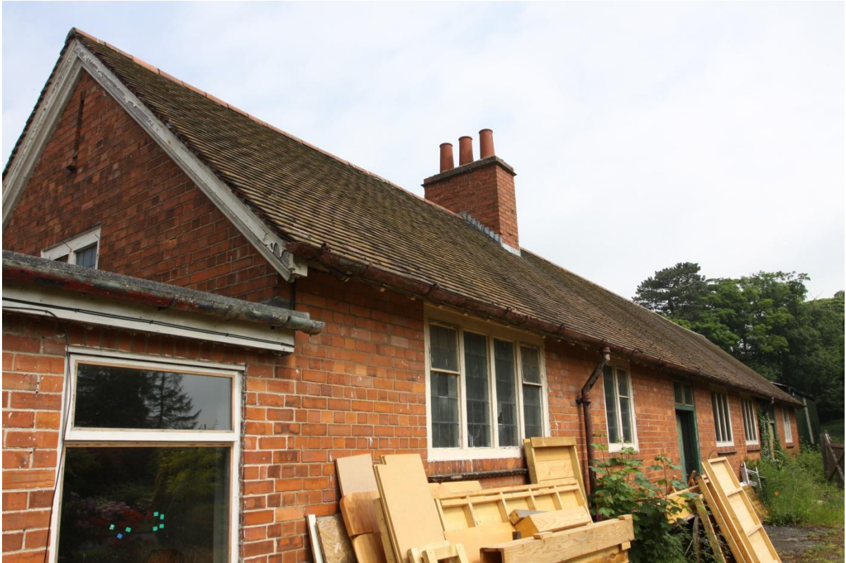
Plate 3 View along the south-eastern elevation, view north-east.
