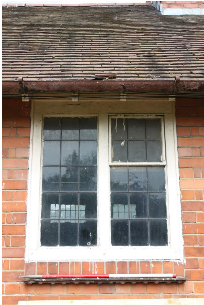
Plate 4 Detail of window in south-eastern elevation of Unit B, view north-west.
