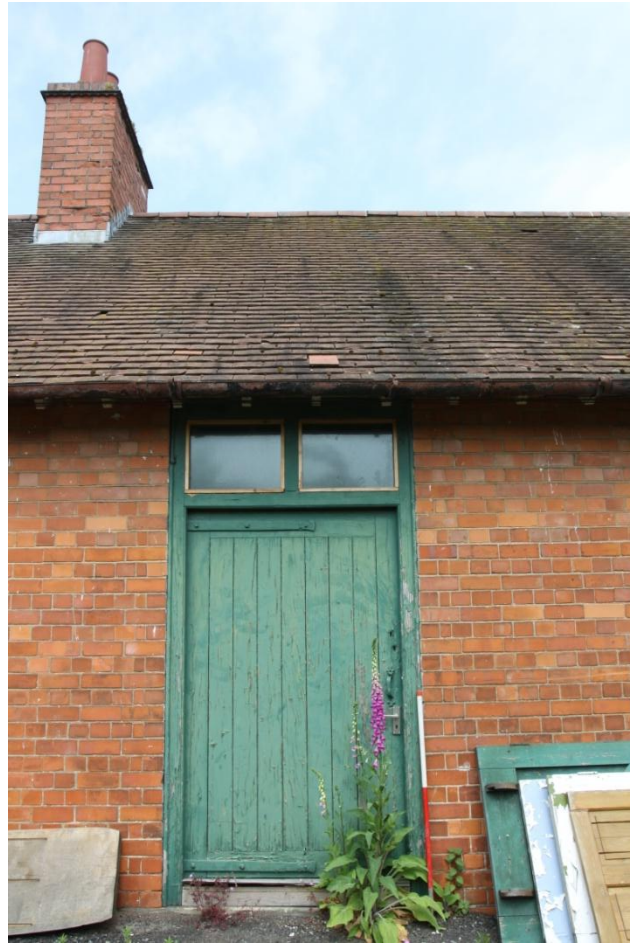
Plate 5 External view of the doorway in Unit C, view north-west.
