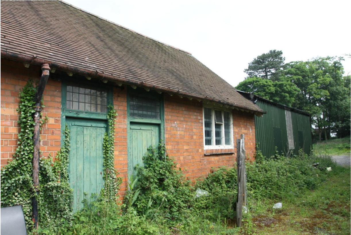
Plate 8 View of the south-eastern elevation of Unit D, looking north-east.
