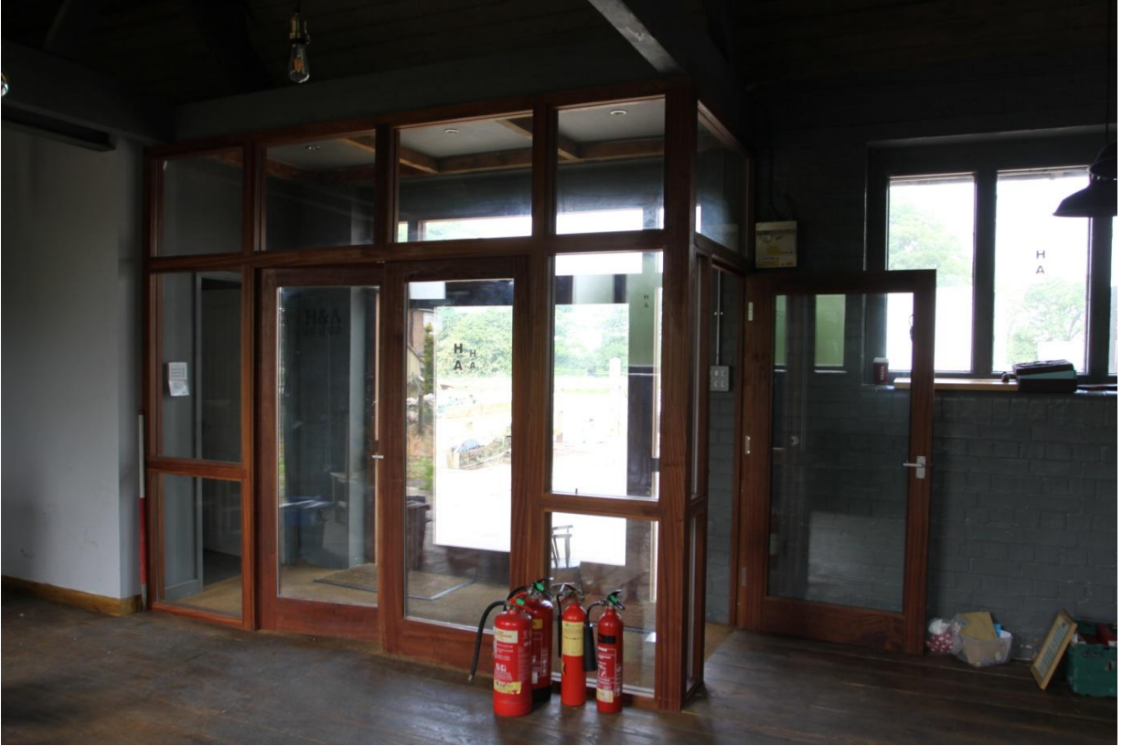
Plate 19 Modern lobby within Unit C, view west.
