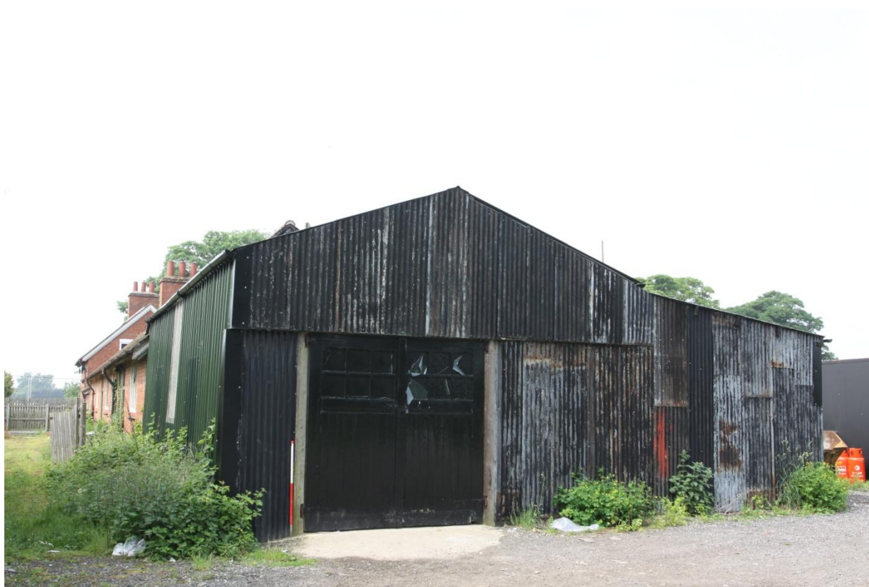
Plate 2 Unit E, view south-west.
