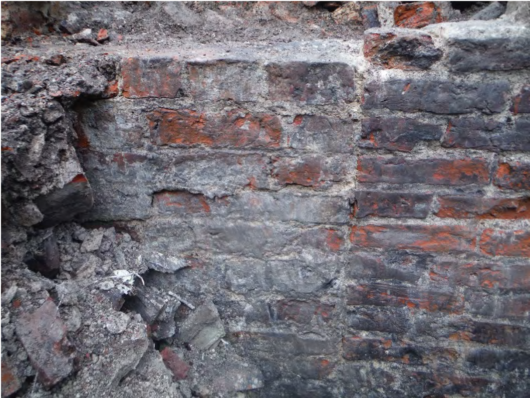
Plate 3 Possible blocked up entrance in wall C102, facing north-west
