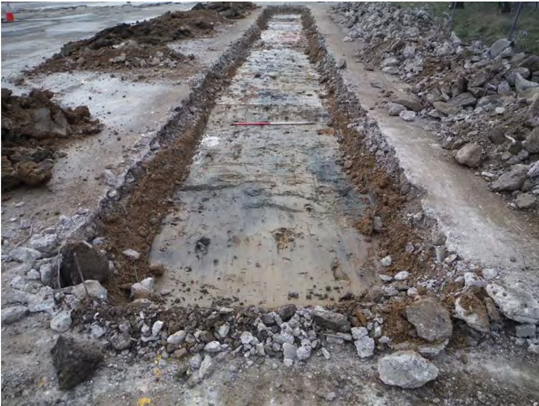
Plate 1 Trench 1, view west
