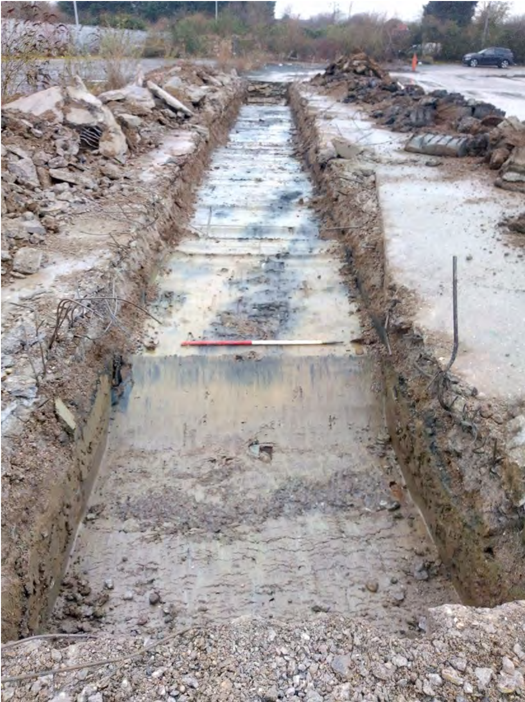
Plate 3 Trench 4, view west
