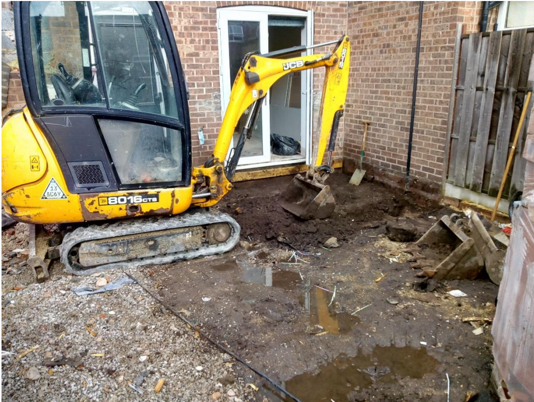
Plate 1 Pre-excitation footing east of existing building looking north west.
