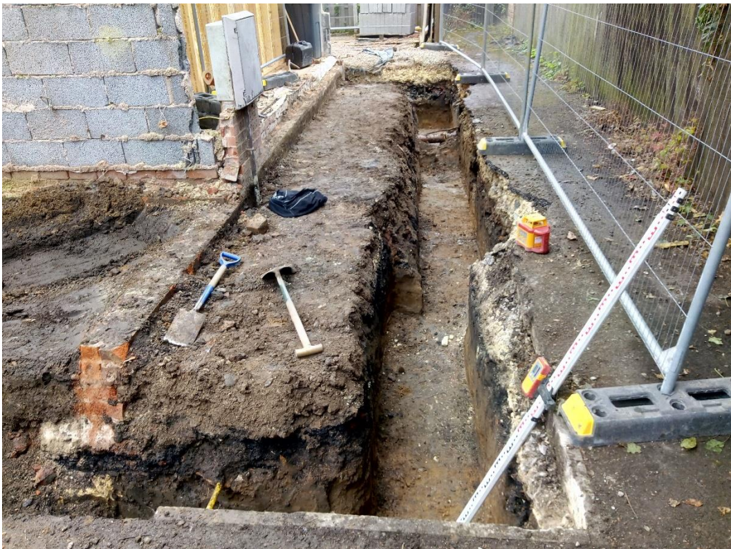
Plate 4 Footings to the south of existing building, looking east.
