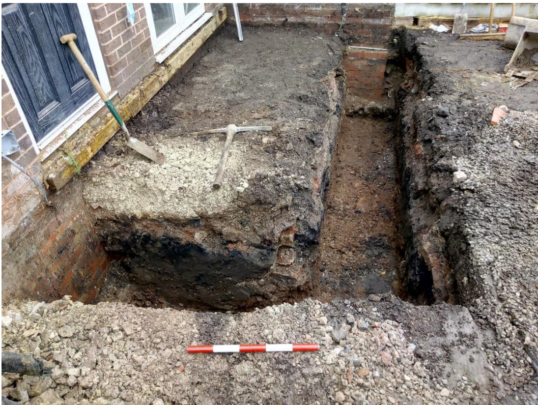
Plate 2 Post-excitation foundation to east of existing building, looking north, 0.5m scale.
