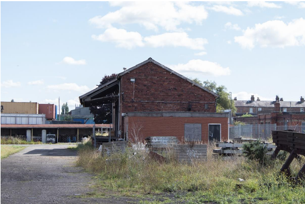
Plate 2: West elevation of the Locks Building
