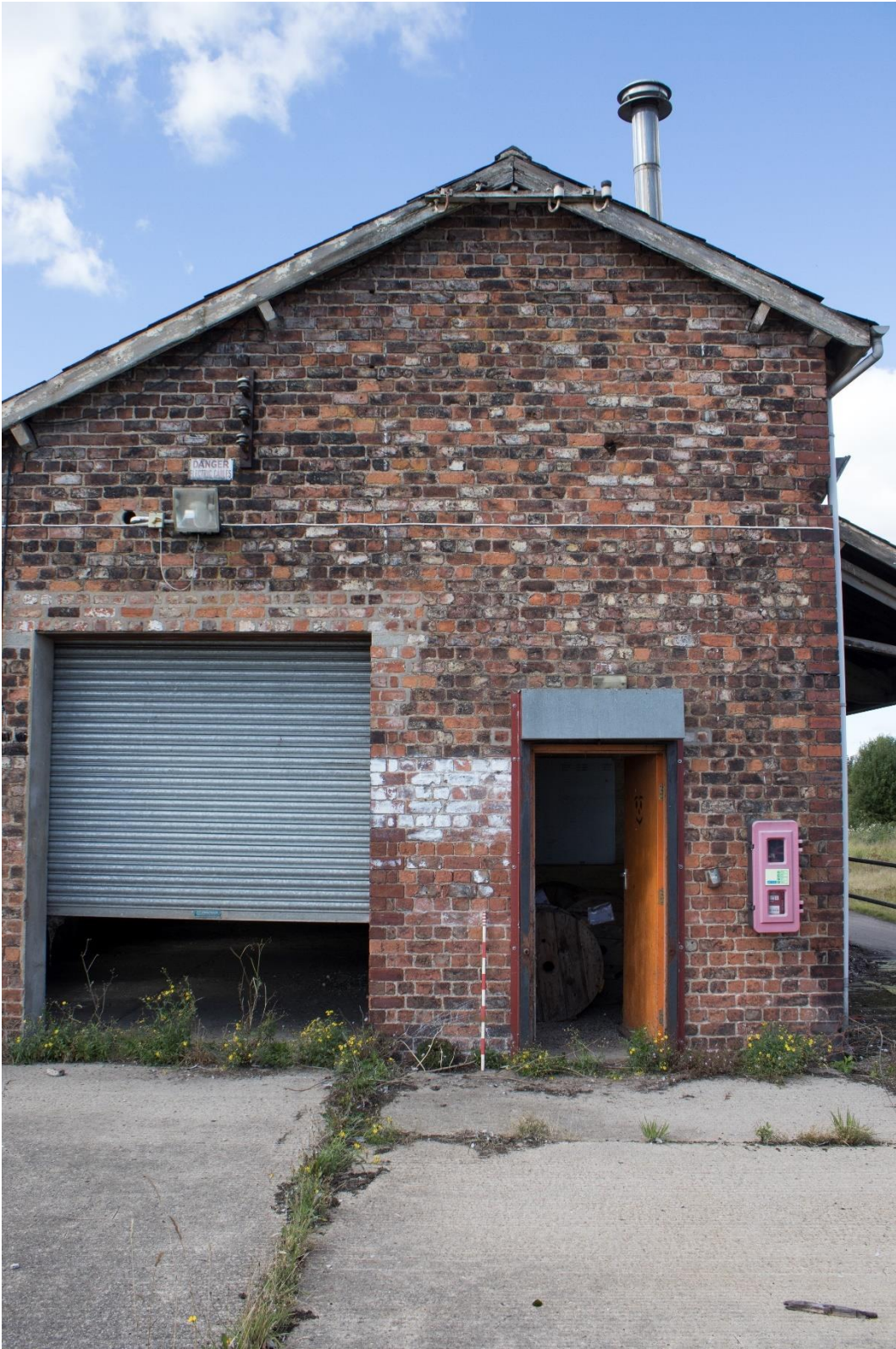
Plate 20: East elevation of the Locks Building, 1m scale
