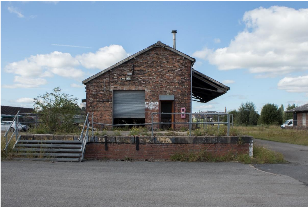
Plate 18: East elevation of the Locks Building, 1m scale
