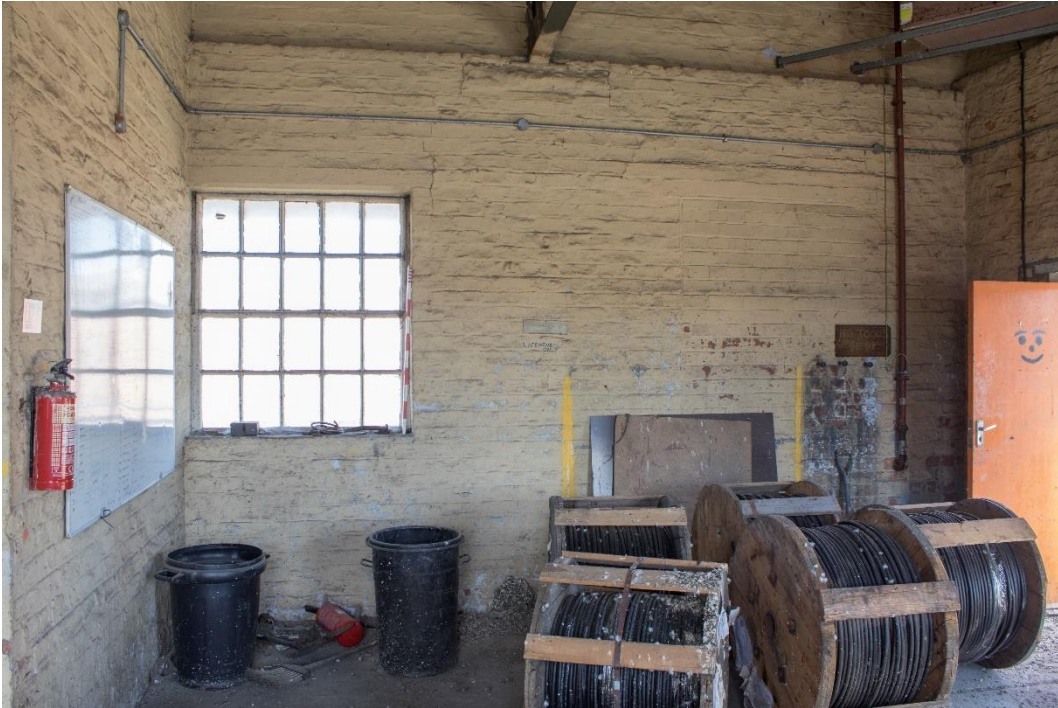
Plate 27: Interior view of north wall and brick partition, 1m scale
