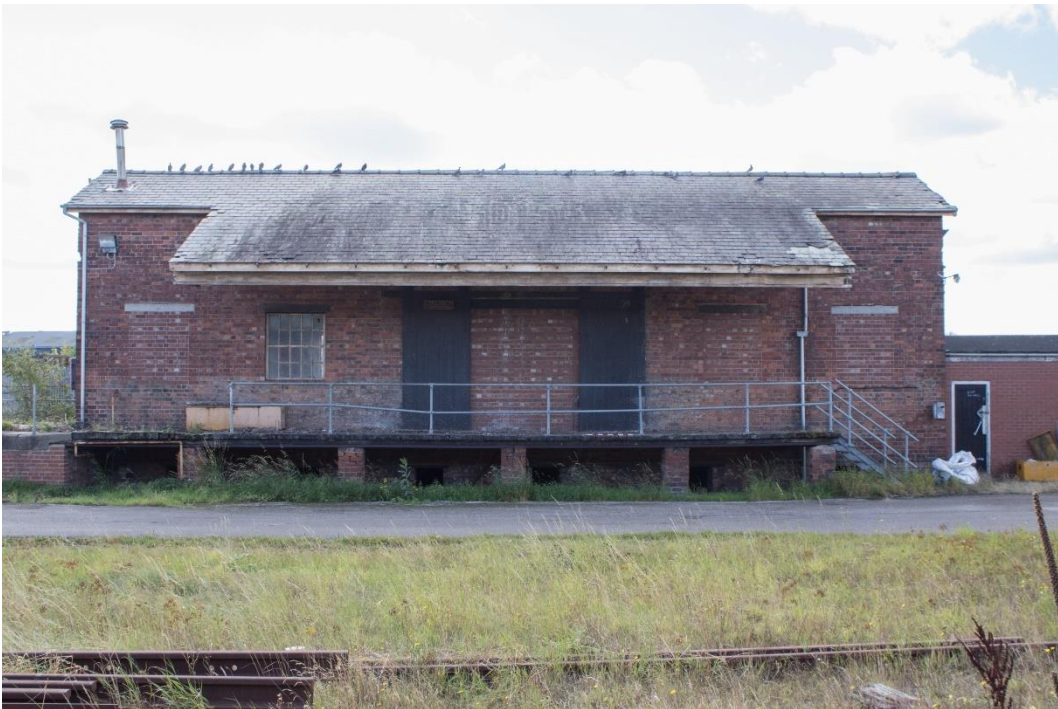
Plate 13: North elevation of the Locks Building, 1m scale
