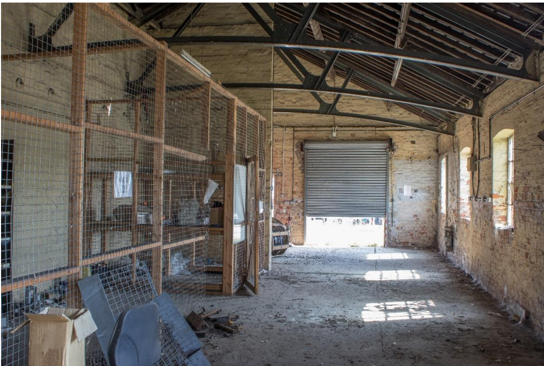
Plate 22: Interior of the Locks Building, view east
