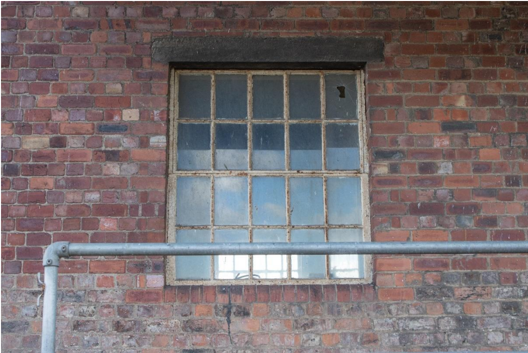
Plate 17: Window in north elevation
