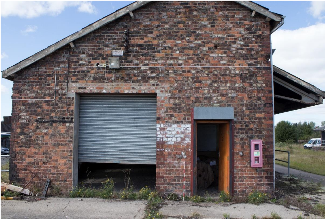
Plate 19: East elevation of the Locks Building, 1m scale
