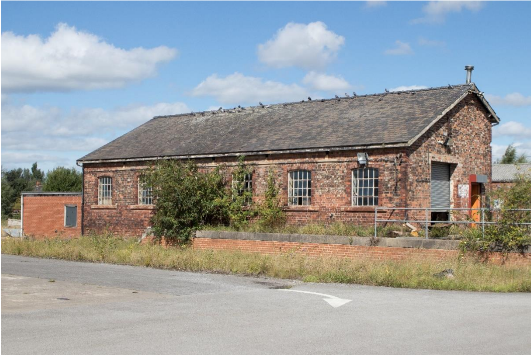
Plate 7: South and east elevations of the Locks Building
