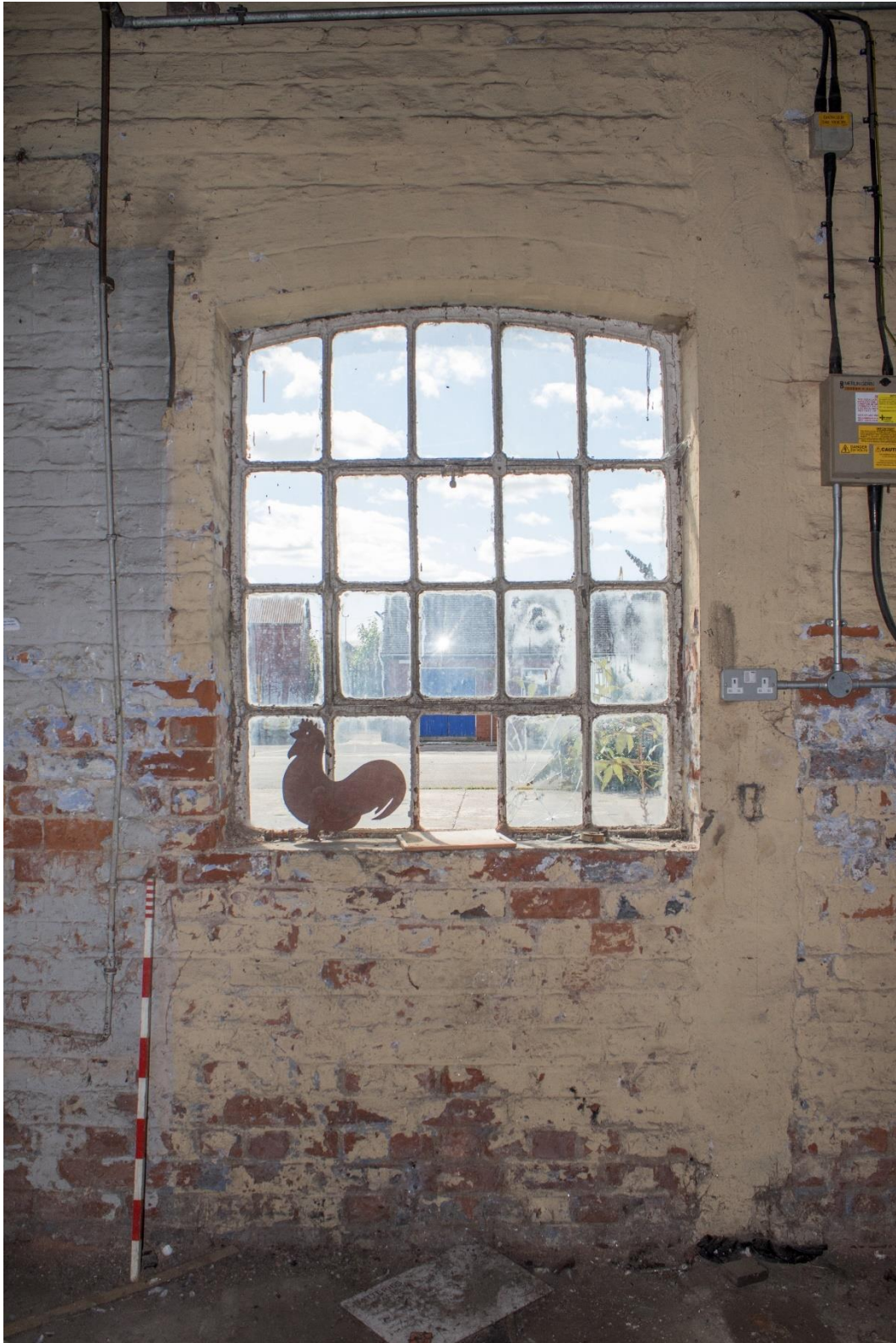
Plate 26: Interior view of window in south wall, 1m scale
