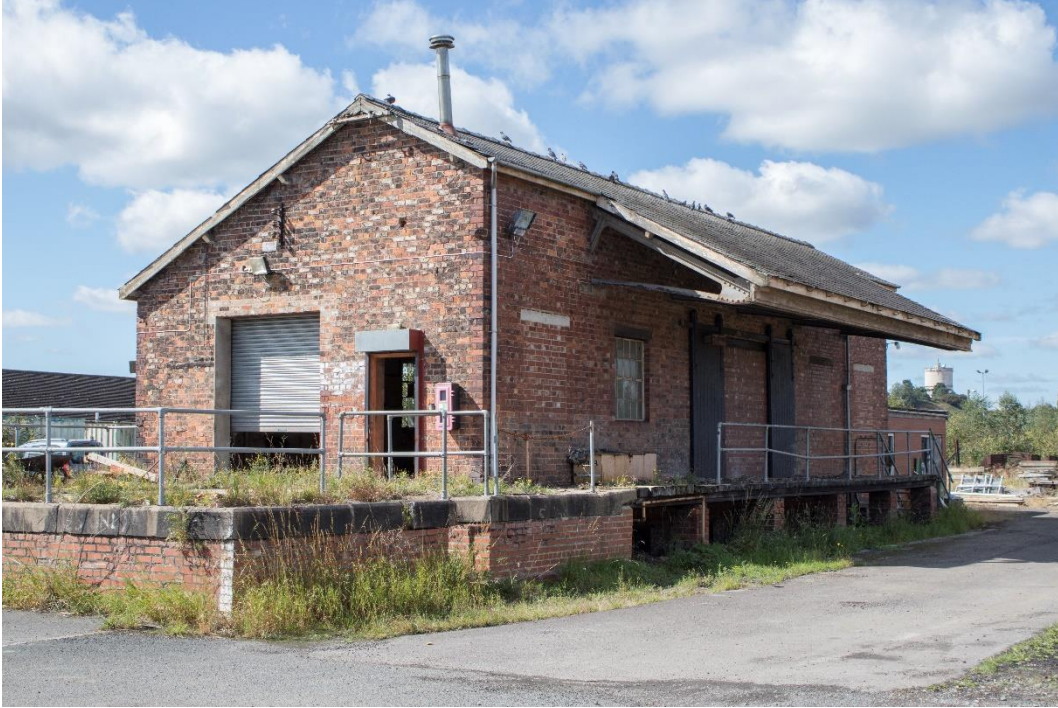
Plate 5: North and east elevations of the Locks Building
