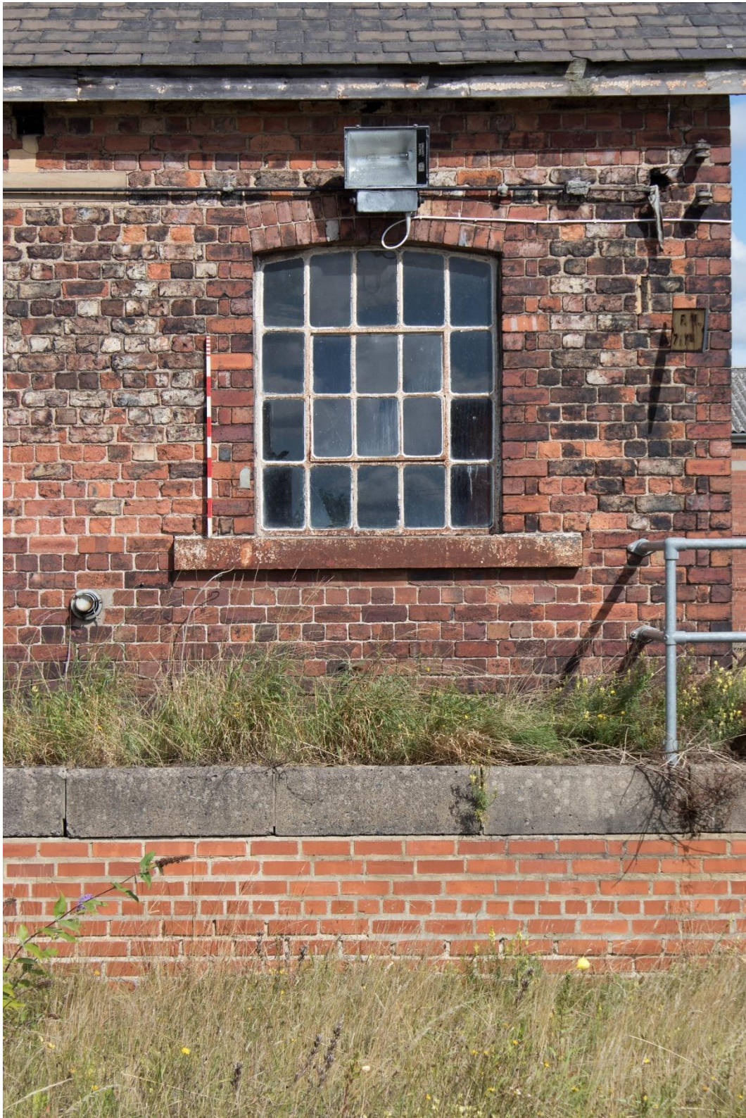
Plate 9: Window in south elevation, 1m scale
