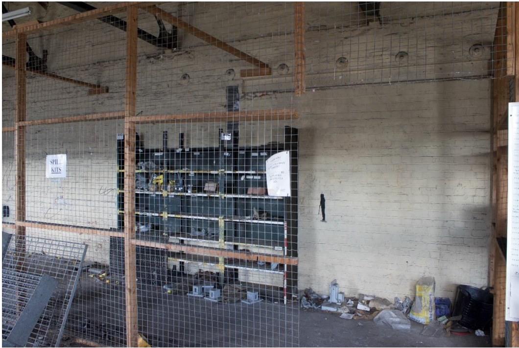
Plate 29: Interior view of north wall showing blocked doorways, 1m scale
