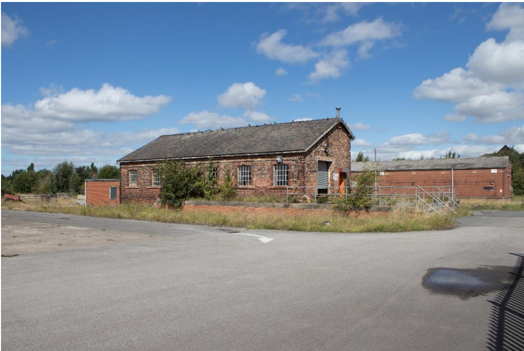
Plate 6: South and east elevations of the Locks Building
