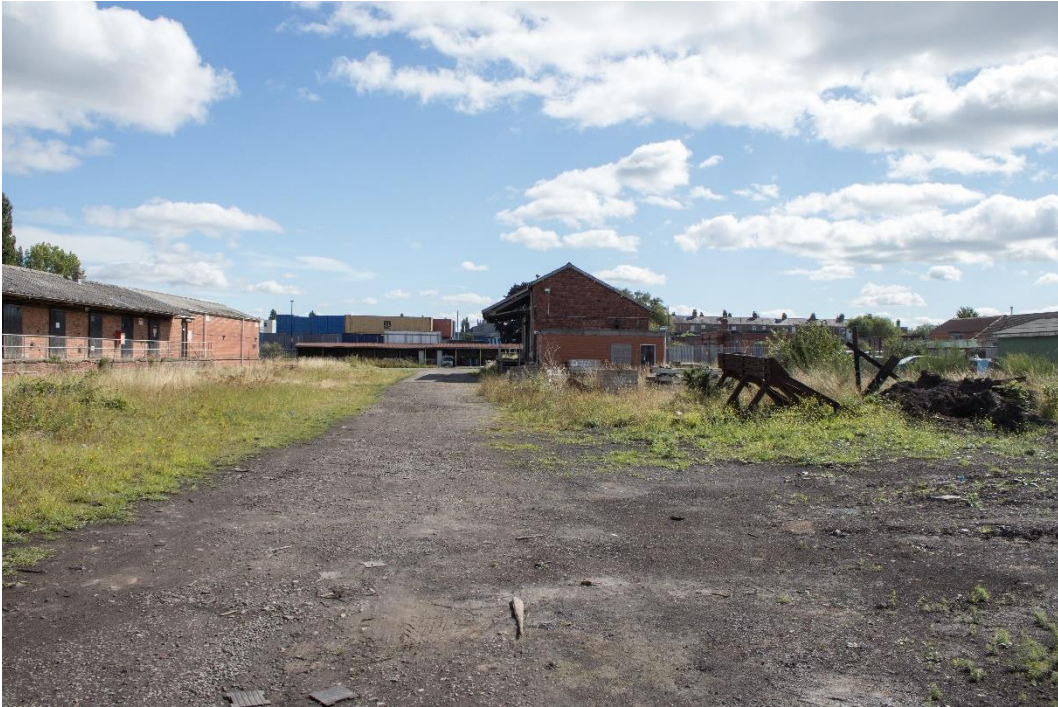
Plate 1: West elevation of the Locks Building
