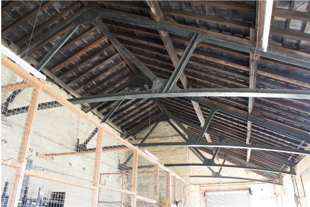
Plate 23: View of the steel roof trusses, looking east
