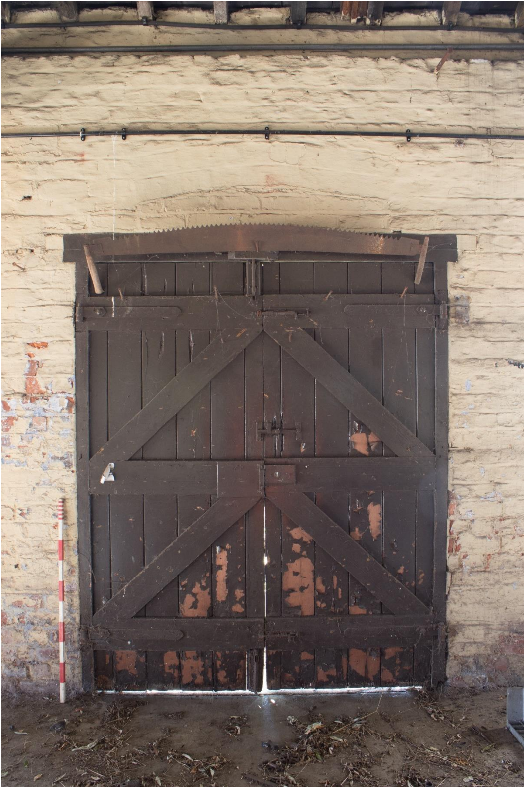
Plate 25: Double doorway with brick arch lintel in south wall, 1m scale
