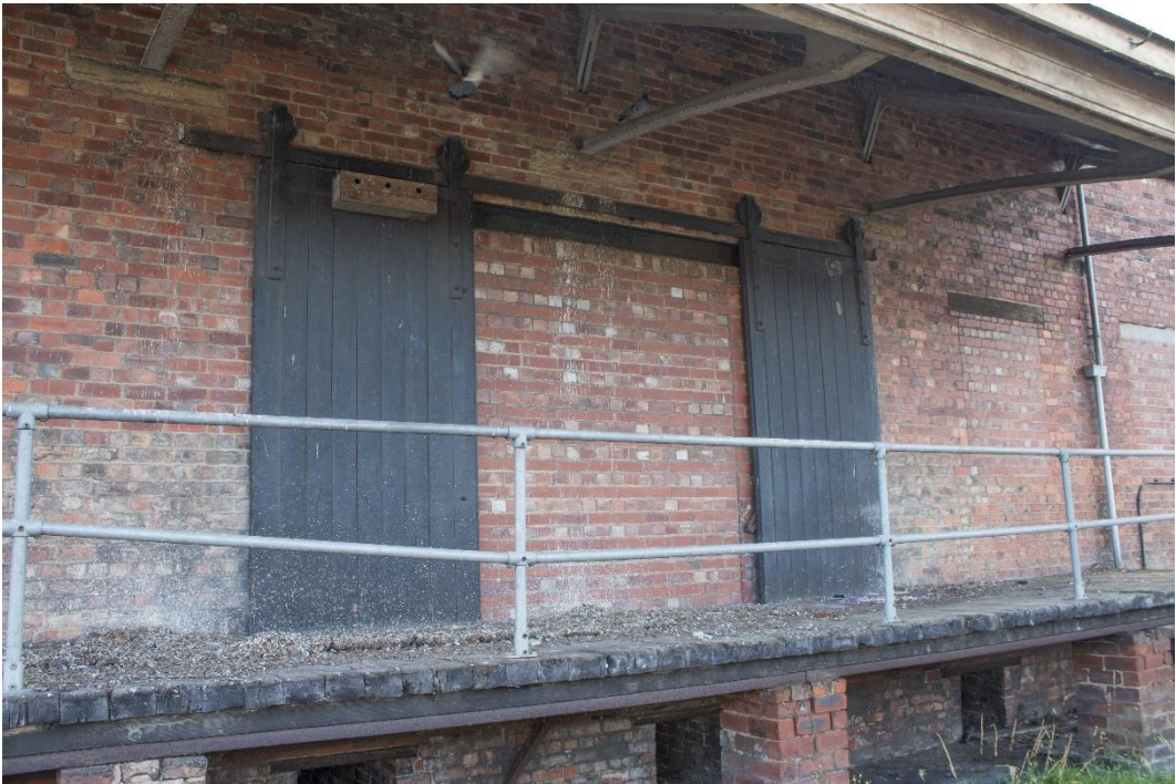
Plate 16: Doorways under canopy on north elevation
