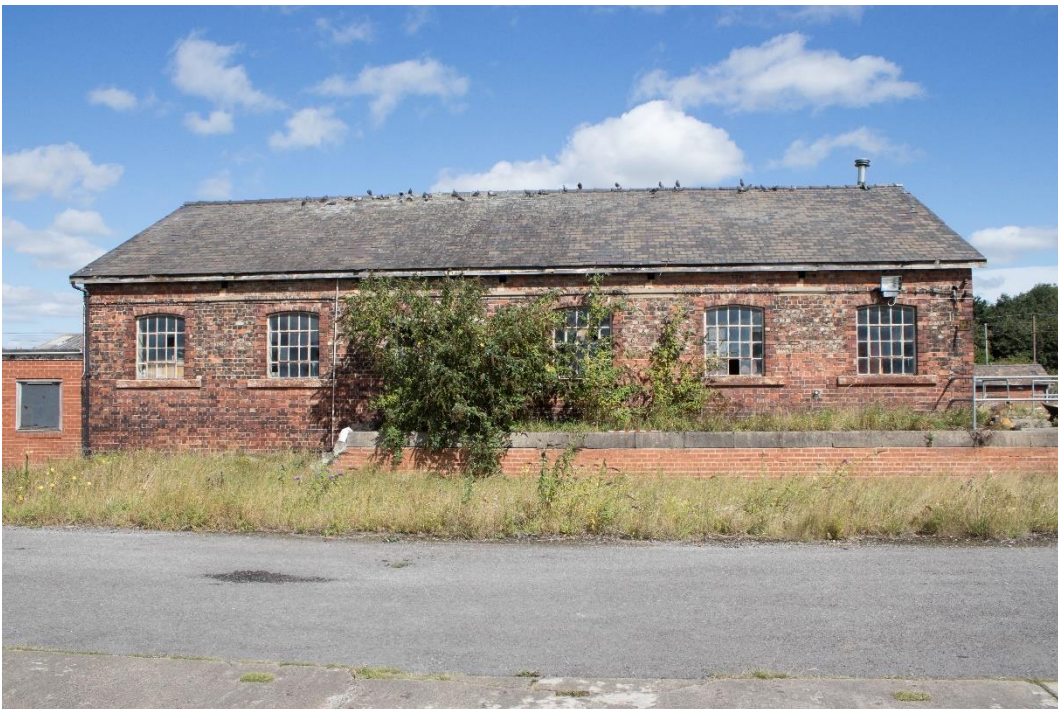
Plate 8: South elevation of the Locks Building
