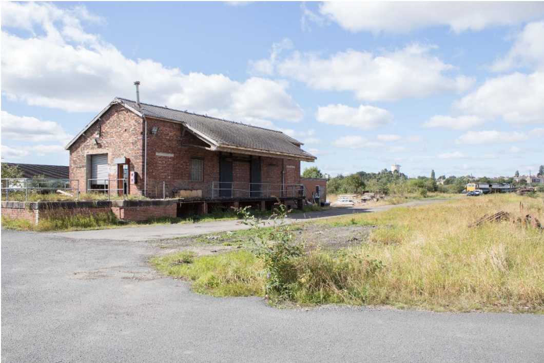
Plate 4: North and east elevations of the Locks Building
