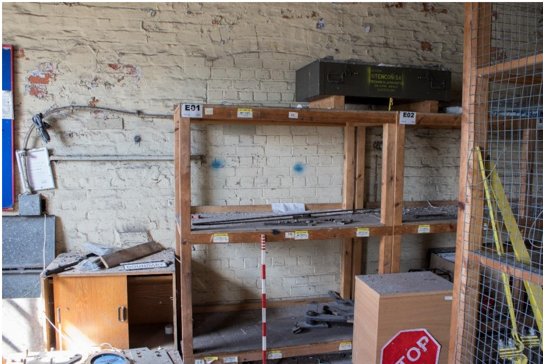
Plate 24: Blocked doorway in west wall, 1m scale
