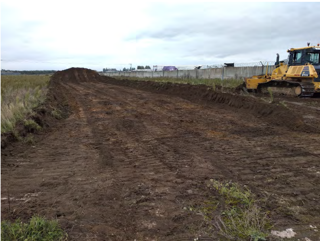
Plate 2 General view of site during topsoil strip.
