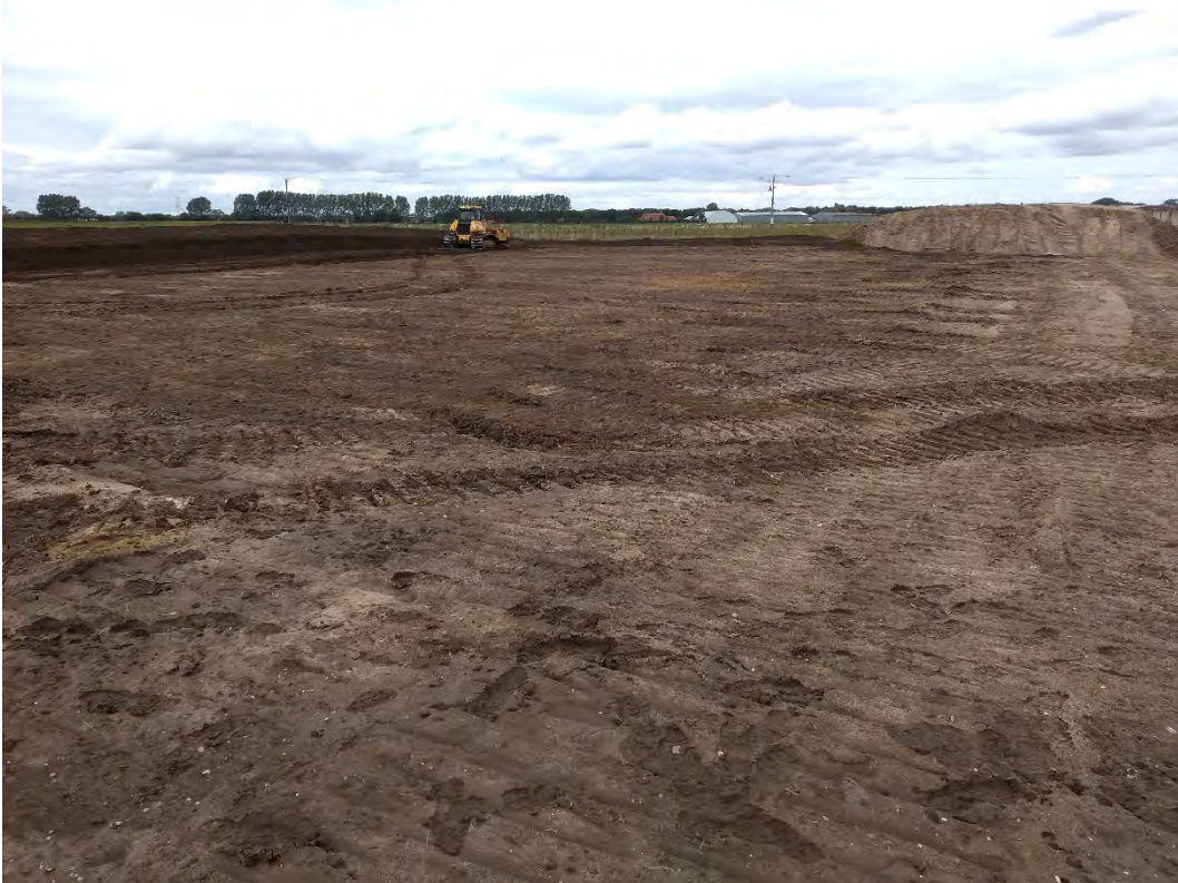
Plate 1 General view of site after topsoil strip.
