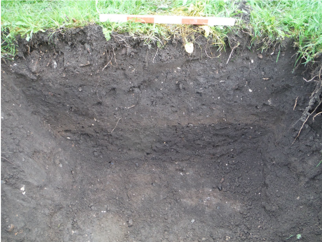
Plate 3 Test pit 3, looking south. Scale 0.5m
