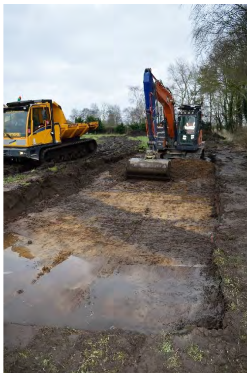
Plate 2 Machining at the southern end of Area A
