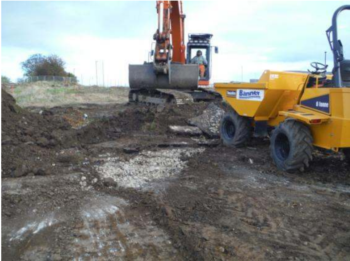
Plate 2. Exposing heavily disturbed deposits in the south-western area of the development area.
