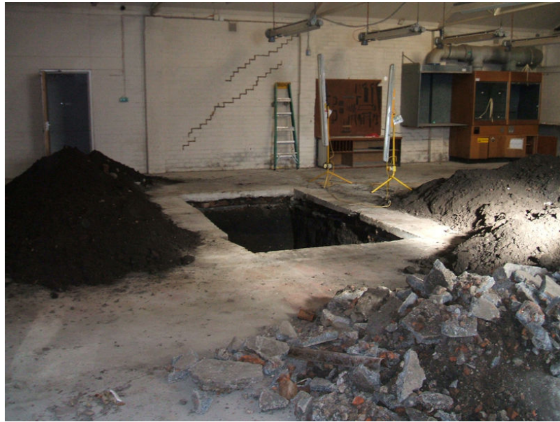
Plate 4 Interior view showing trench and light conditions, looking north
