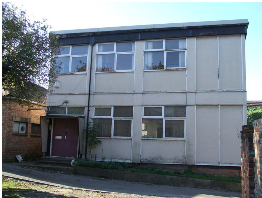
Plate 3 Terrapin building, showing extent of made-ground, looking south-east
