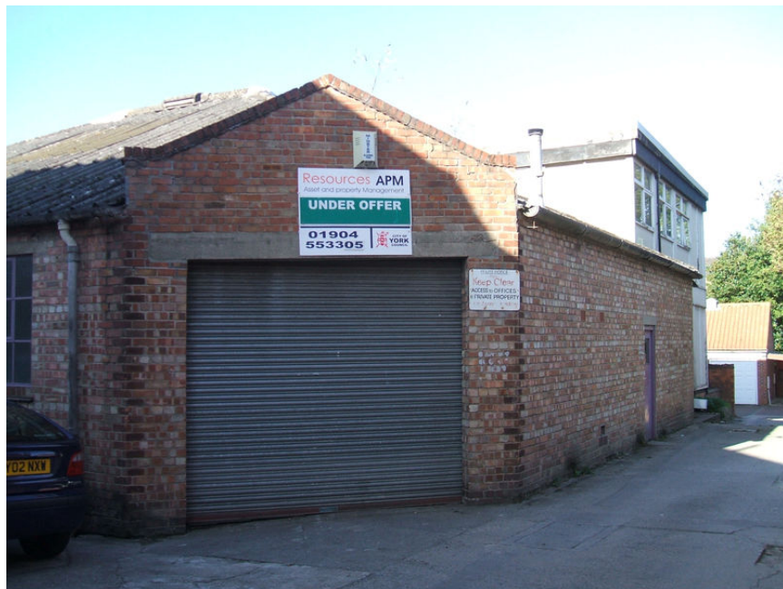
Plate 2 Brick-built laboratory with Terrapin building behind, looking north-west
