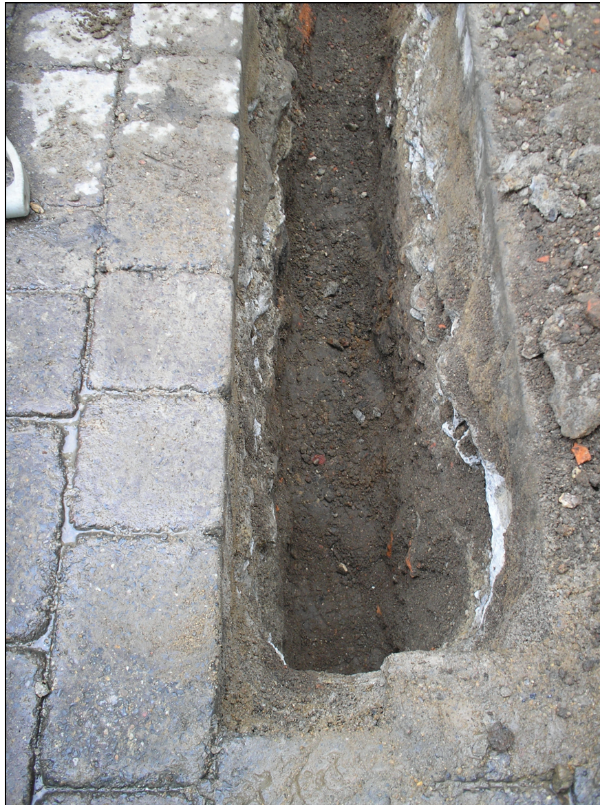
Plate 3 South-west half of July trench, looking north-east
