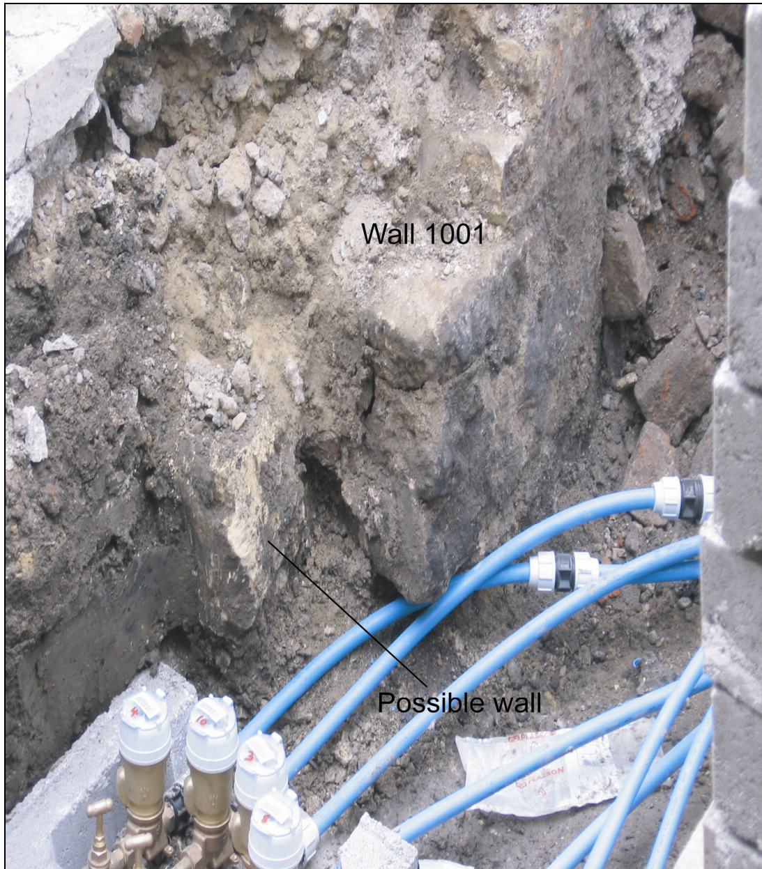
Plate 2 Detail view of wall 1001, looking south-east
