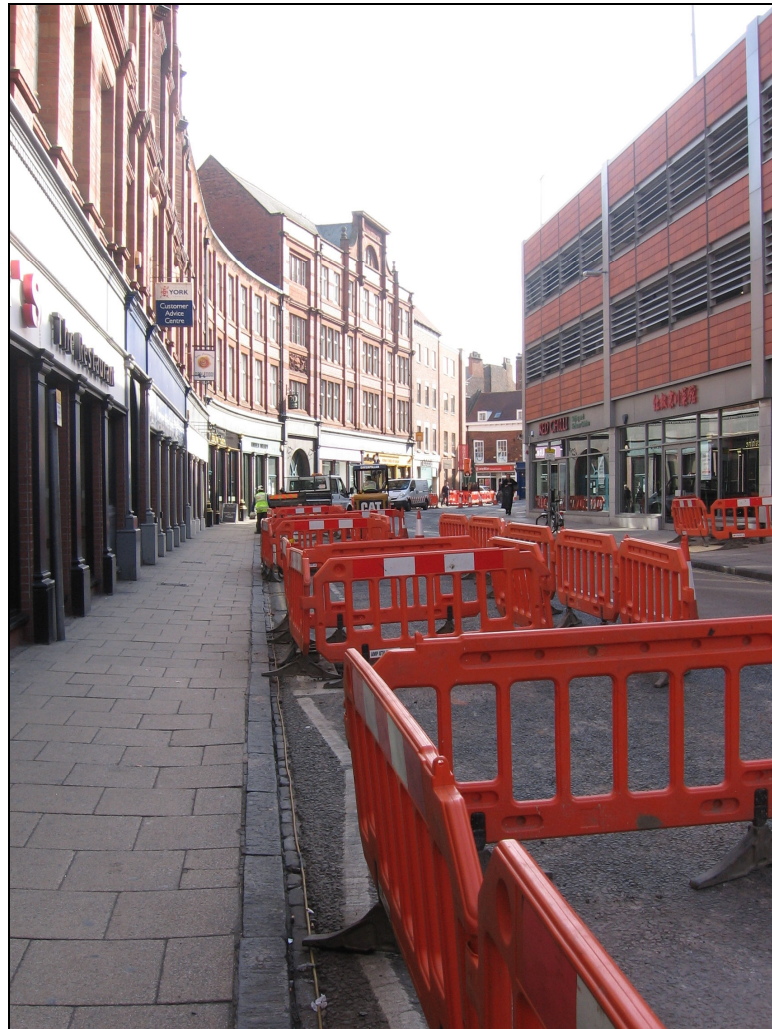
Plate 3 General view of works in progress, looking south
