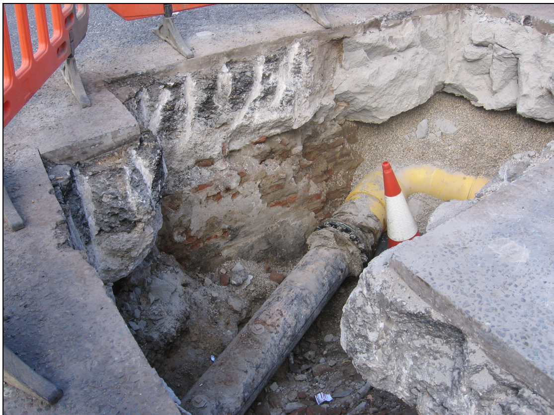
Plate 1 Gas main and wall 1006 in Trench 1, looking north-west
