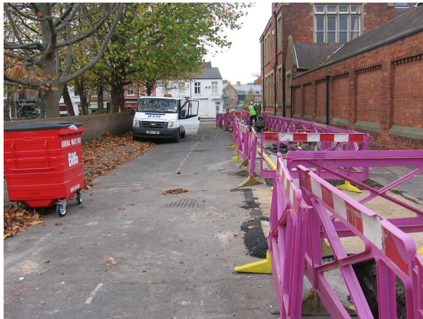
Plate 1 General view of trench along Winterscale Street, looking W
