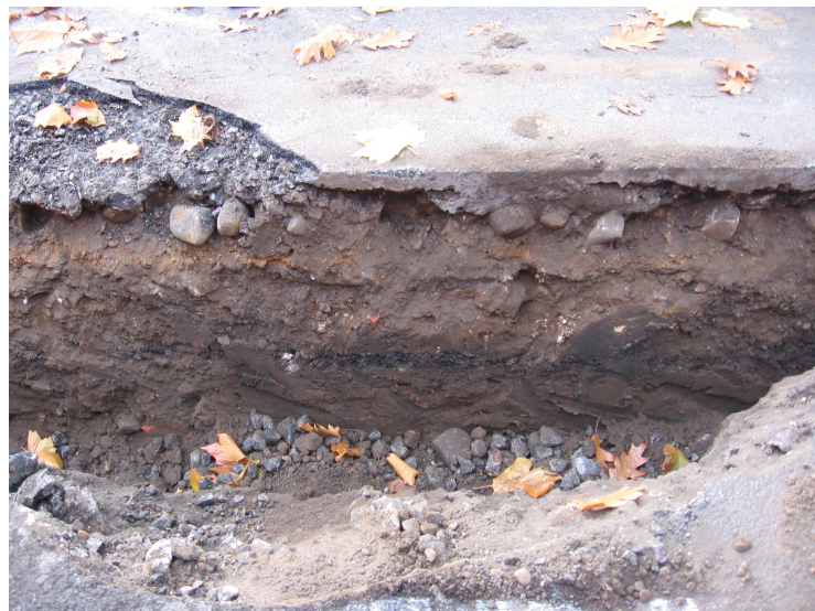
Plate 3 Trench section along central part of trench, looking S
