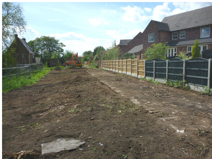
Plate 1 Looking west from eastern end of site with road 1002
