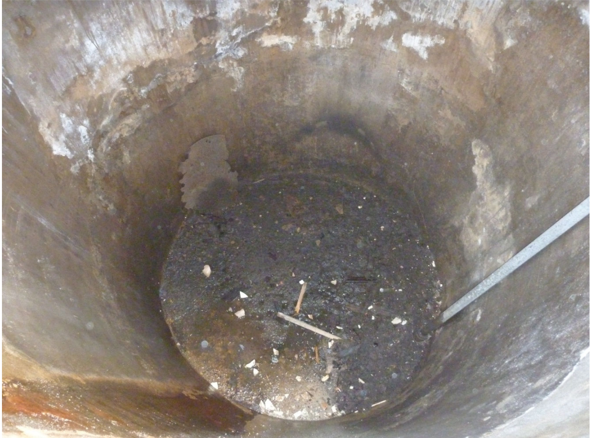
Plate 9 View into ice house chamber through access manhole
