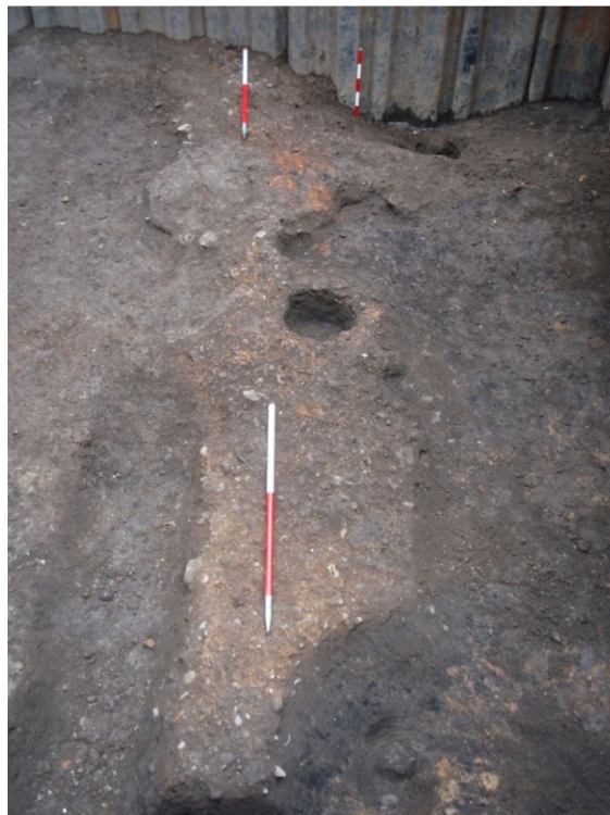
Plate 11 Possible yard surface 1078, looking south-east
