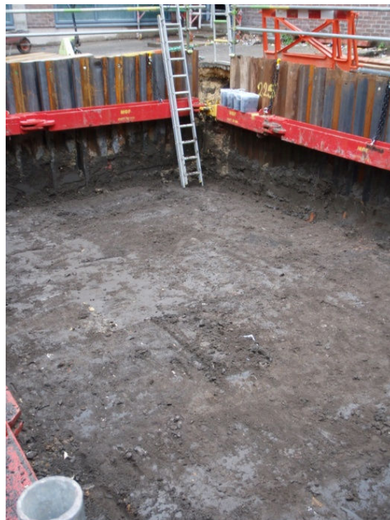
Plate 20 Medieval plough-soils during machine stripping, looking east
