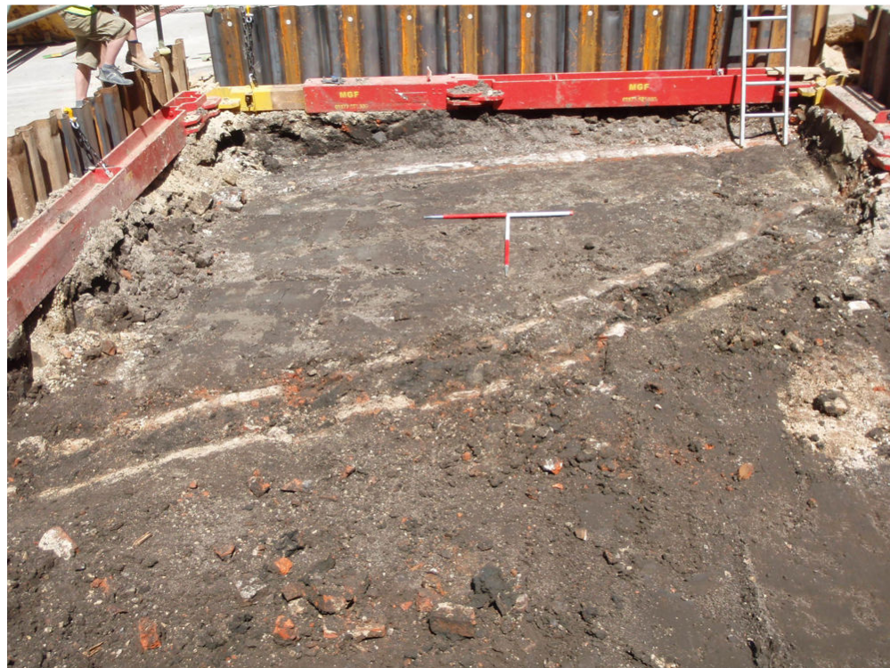
Plate 21 Culvert 1021-1022, looking north-east
