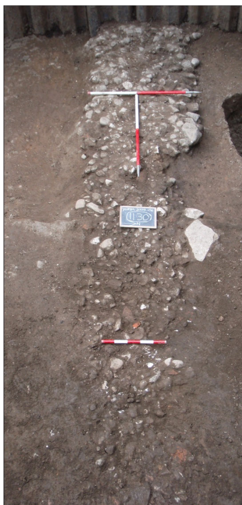
Plate 2 Phase 2 road surface 1130, looking north-west
