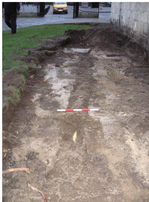
Plate 3 Context 8011 and services trench fill 8007-8, facing south, scale unit 0.1m
