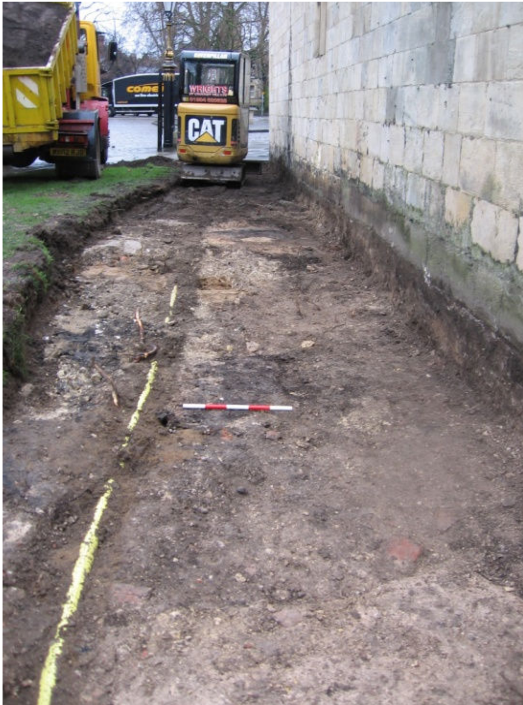
Plate 4 Context 8011 and services trench fill 8007-8 ,facing south, scale unit 0.1m
