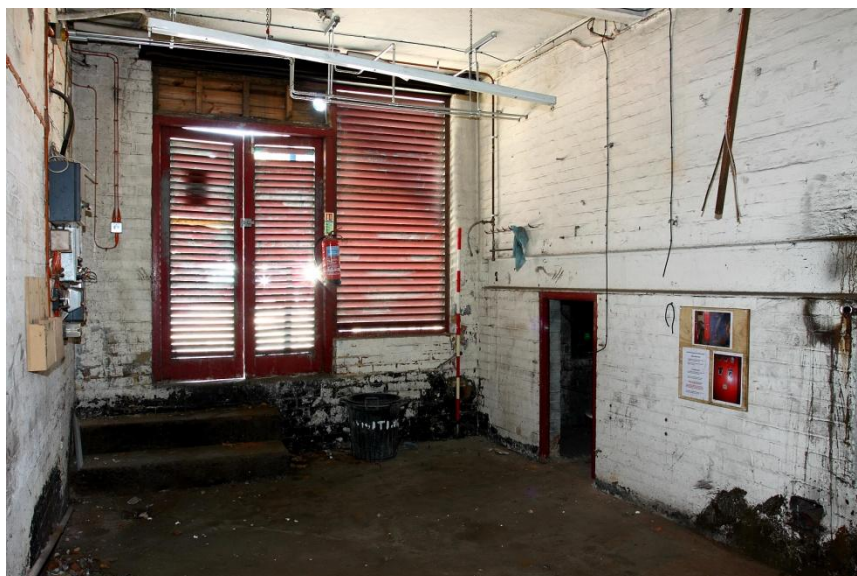
Plate 8 Boiler room, looking NE
