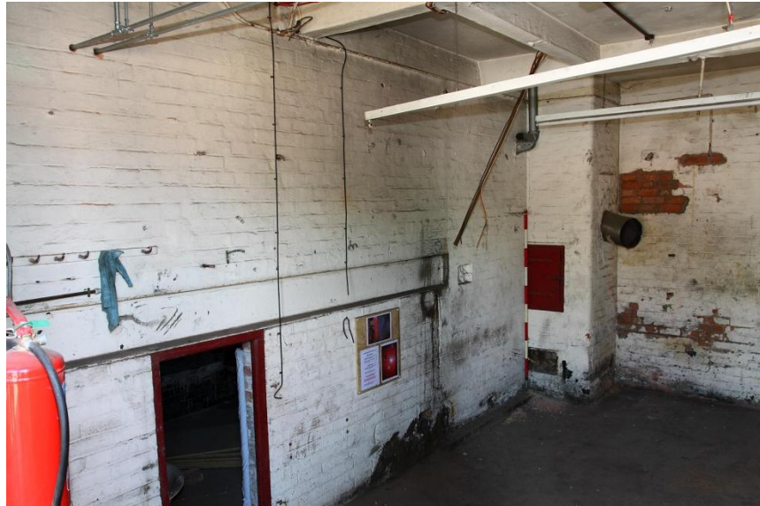
Plate 7 Boiler room, looking S
