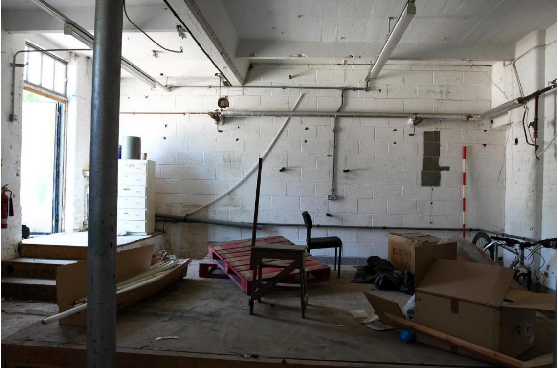
Plate 5 Plant room, looking SE
