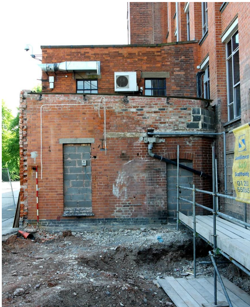
Plate 3 NW facing elevation
