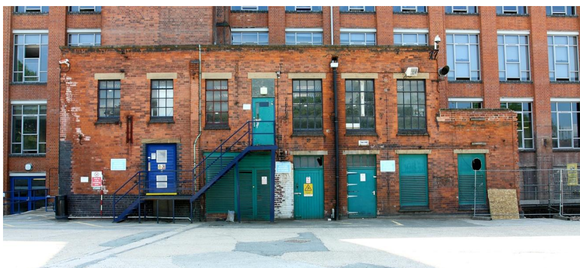
Plate 2 NE facing elevation
