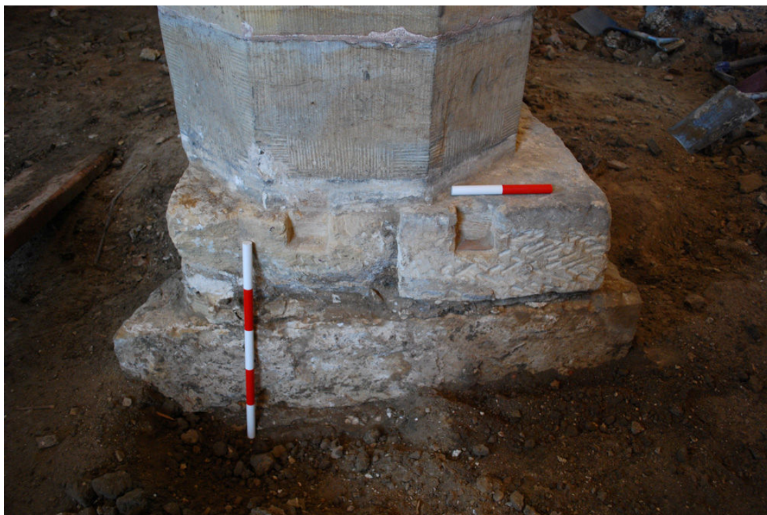
Plate 4 Pier footing 1008 looking north
