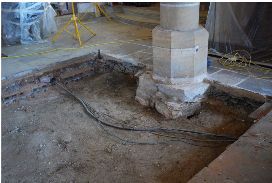
Plate 12 Looking north-east: dwarf walls and sub-floor deposit 1003 with footing 1004
