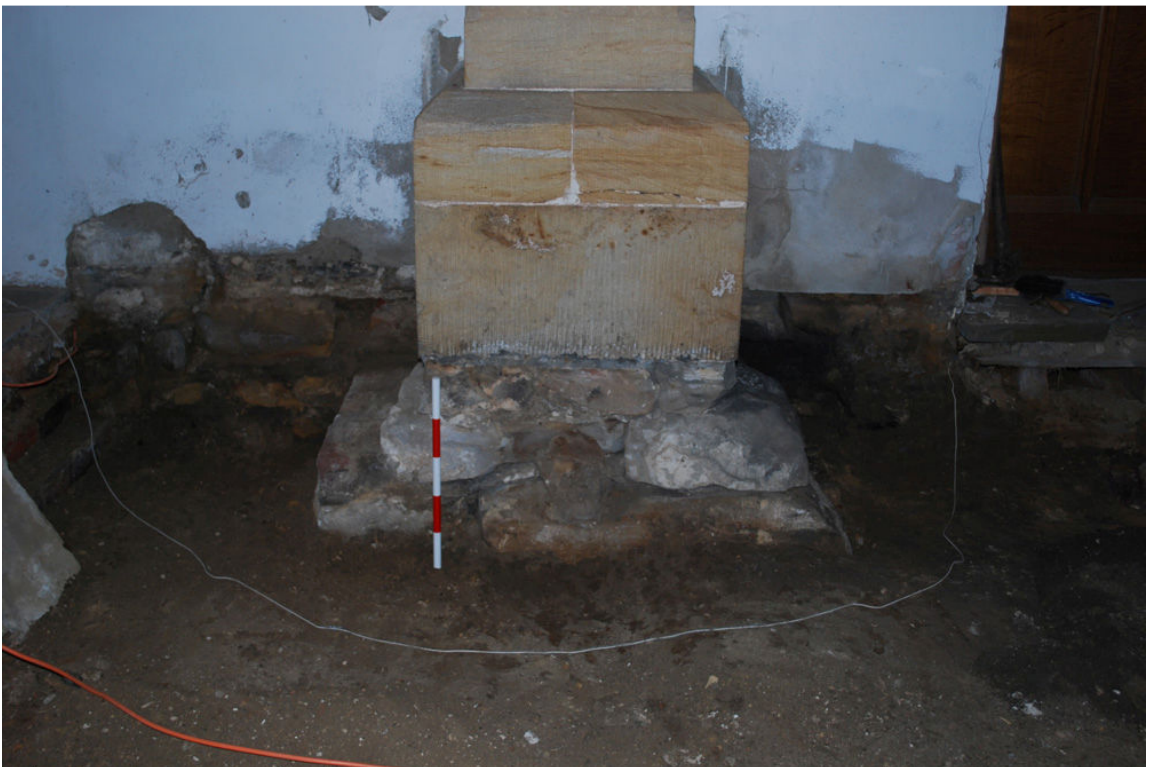
Plate 8 Pier footing 1010 looking west
