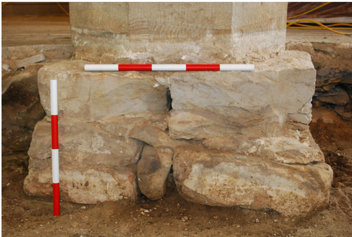
Plate 6 Pier footing 1004 looking east
