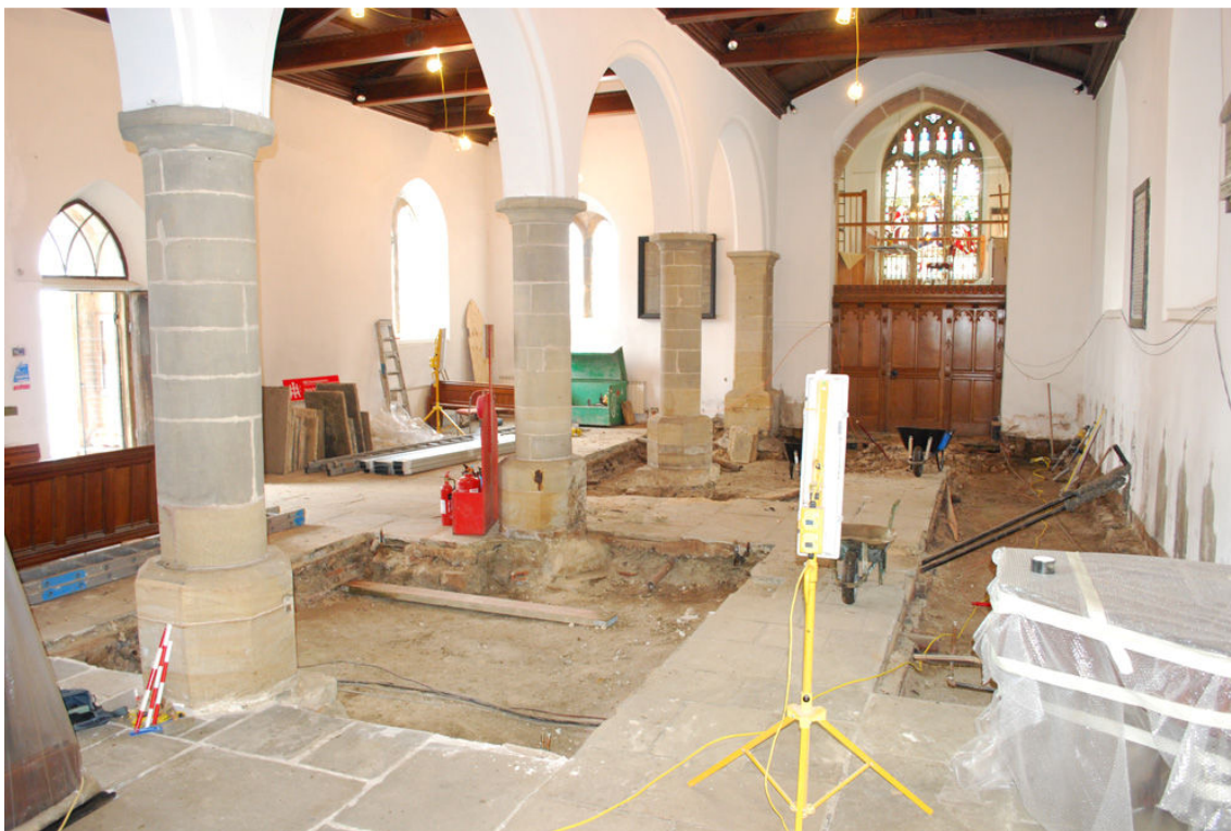
Plate 11 General view looking south-west, showing pier footings and sub-floor deposit 1003
