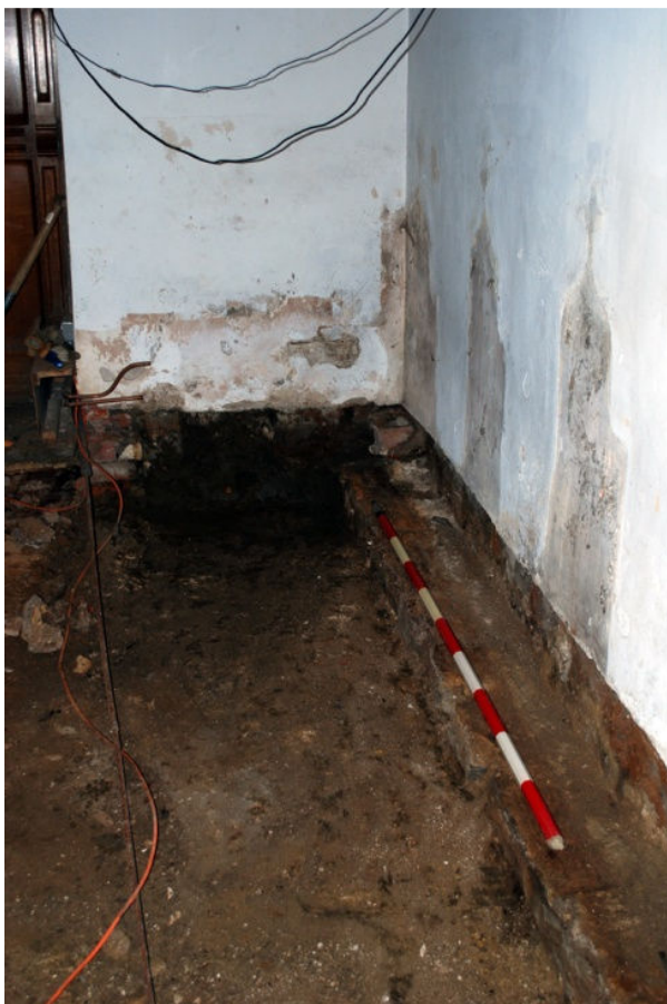
Plate 9 Structure 1012, looking west
