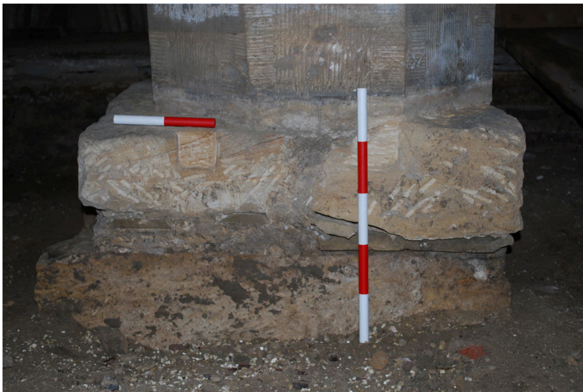
Plate 5 Pier footing 1008 looking south
