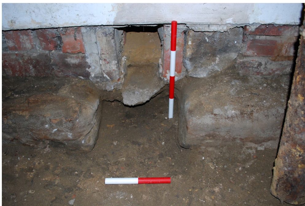
Plate 10 Flue feature 1014 looking north
