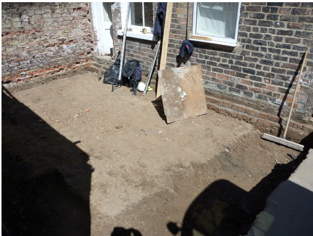
Plate 15 Final view of excavation looking north-west
