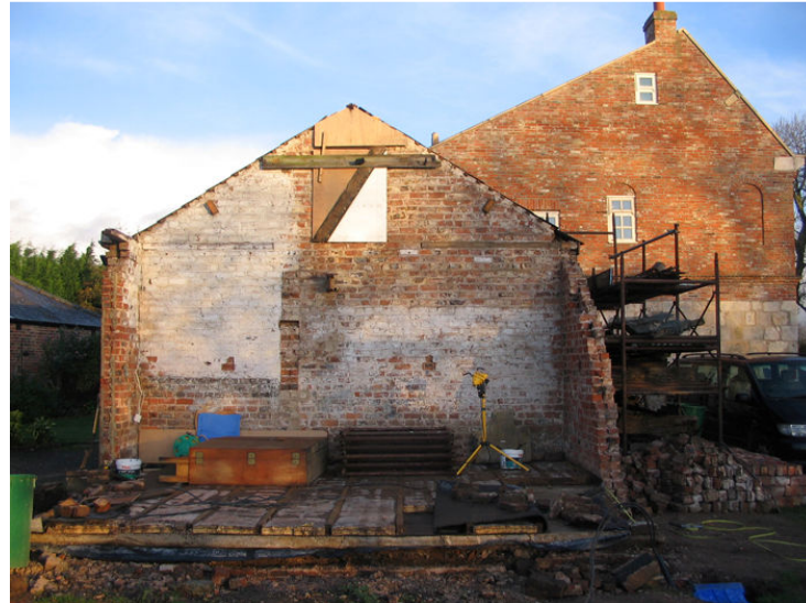
Plate 1 Partly demolished outbuilding, looking north, showing Squirrel Cottage behind
