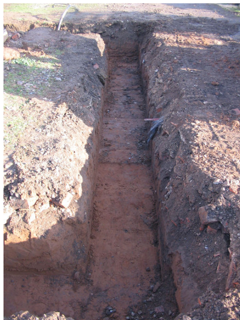
Plate 4 Southern end of foundation trench, looking east
