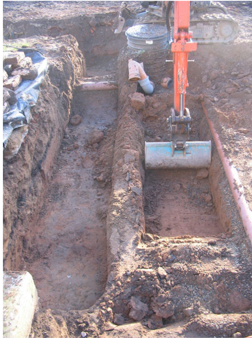
Plate 5 Excavation of stairwell footing, looking south
