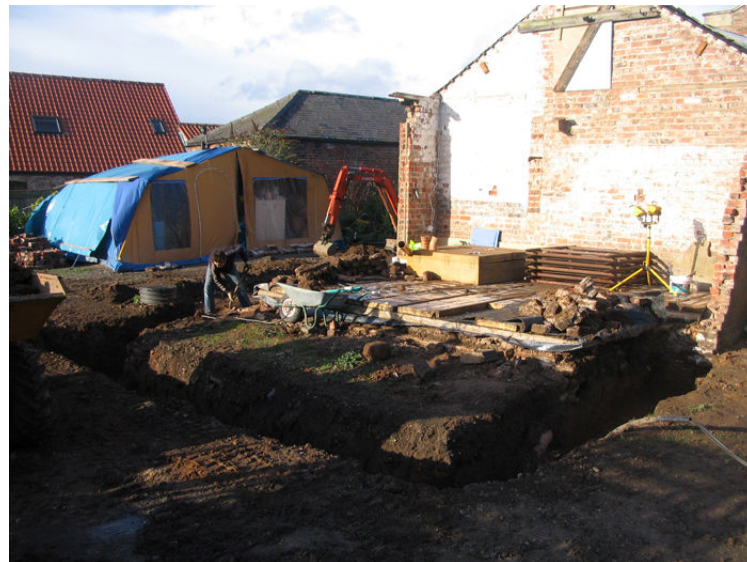
Plate 6 View of completed foundation trench looking north-west
