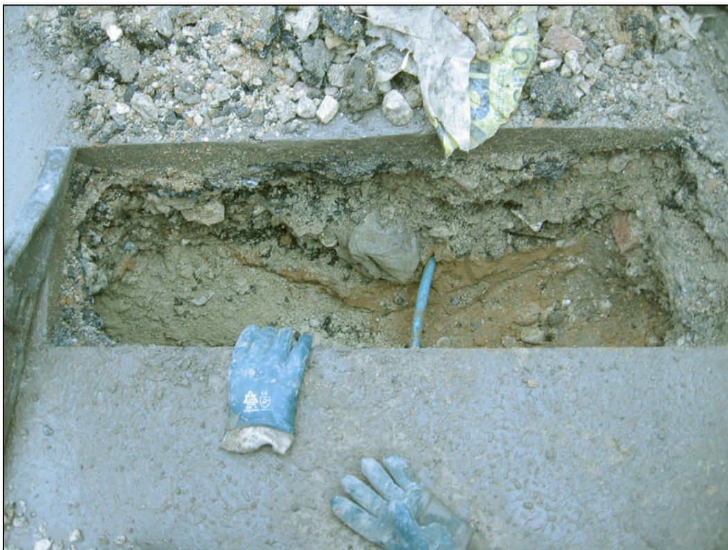
Plate 1 Section 3, looking north-west
