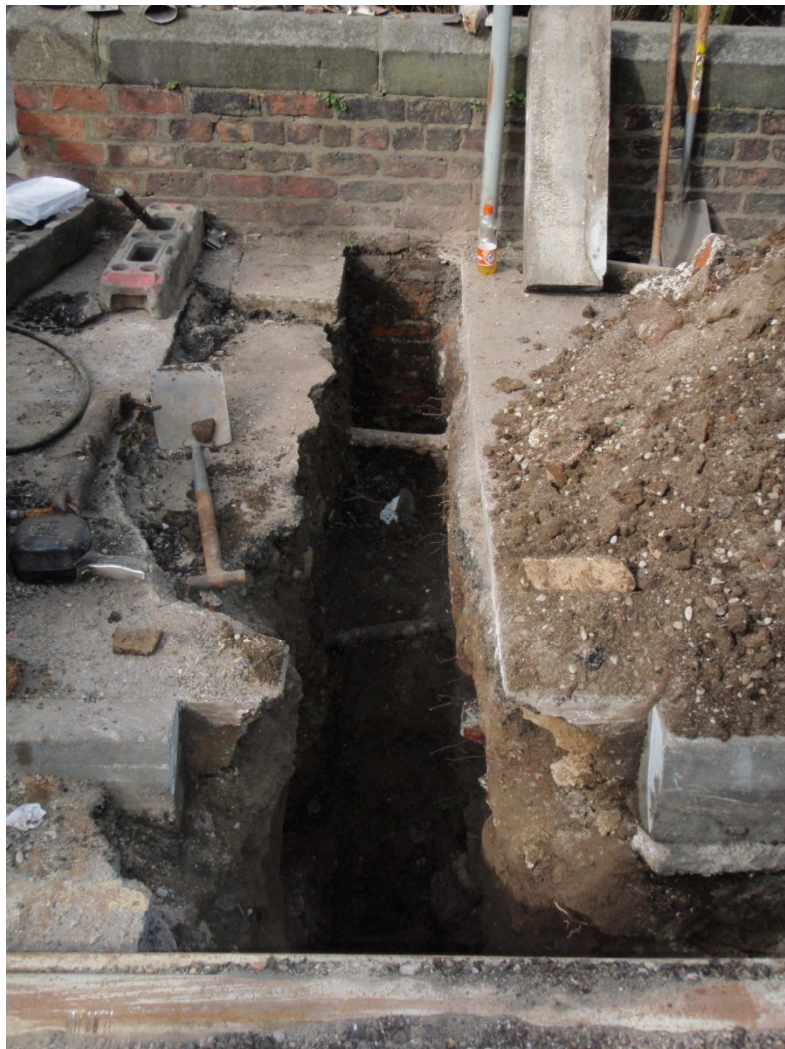
Plate 2 Sewer trench dug through pavement towards churchyard wall
