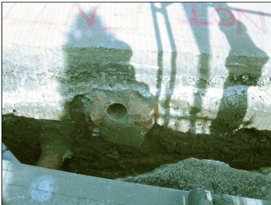
Plate 1 Culvert 1011, looking north-west
