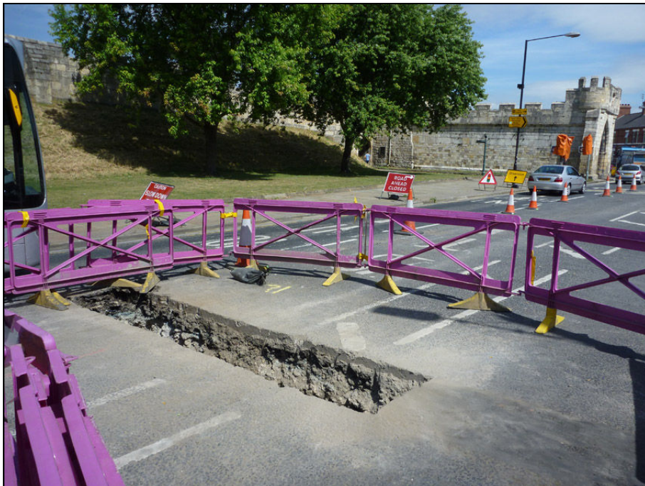
Plate 4 General view of work in Barbican Road, looking north
