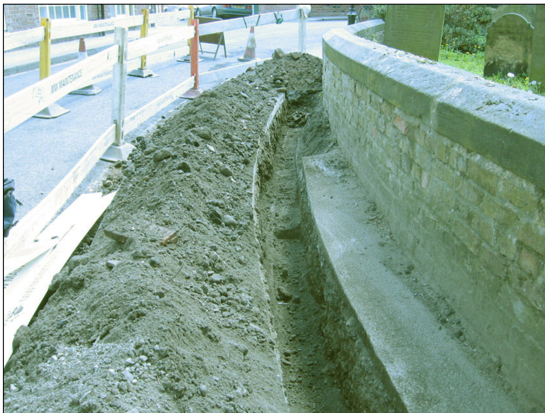
Plate 1 South end of cable trench in Bishophill Junior, looking south
