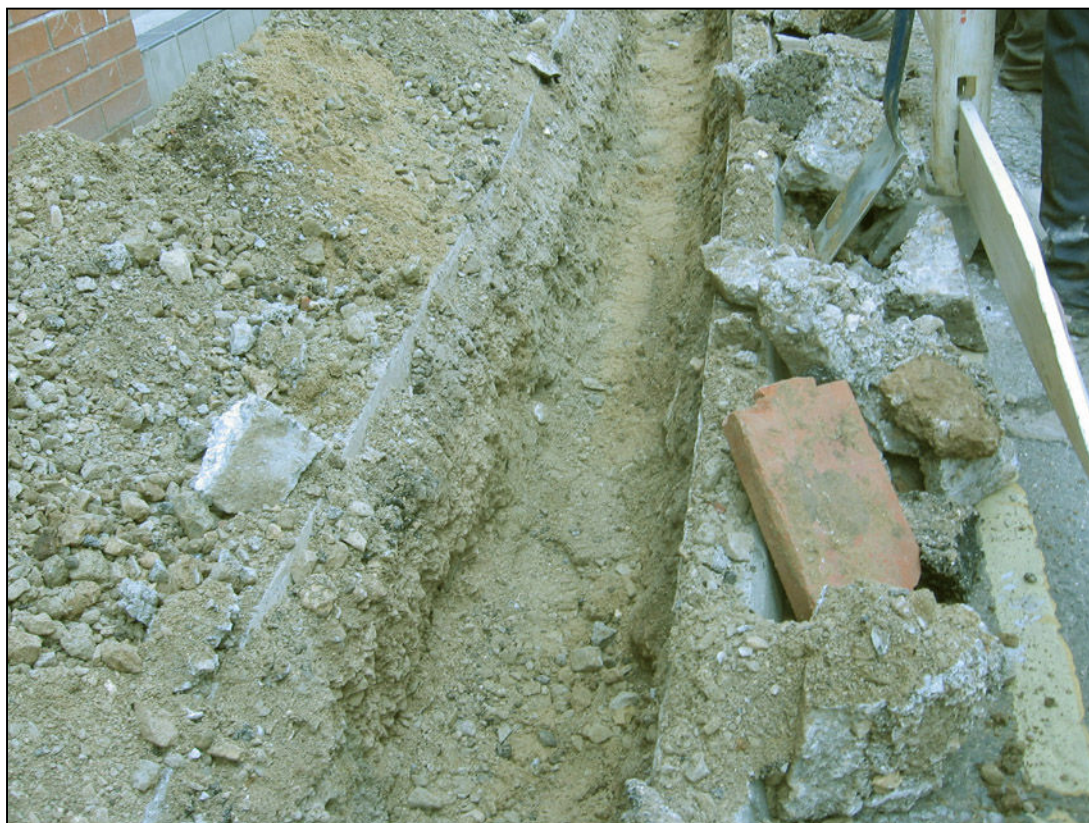
Plate 2 Southern part of cable trench in Fetter Lane, looking south
