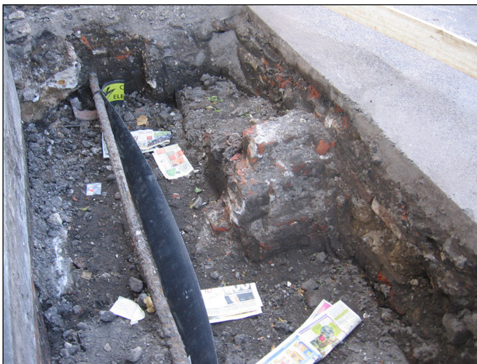
Plate 3 Trench adjacent to Radio York studios, looking south-east
