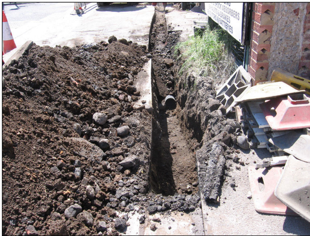
Plate 2 The trench in the central part of Bootham Row, looking south-west
