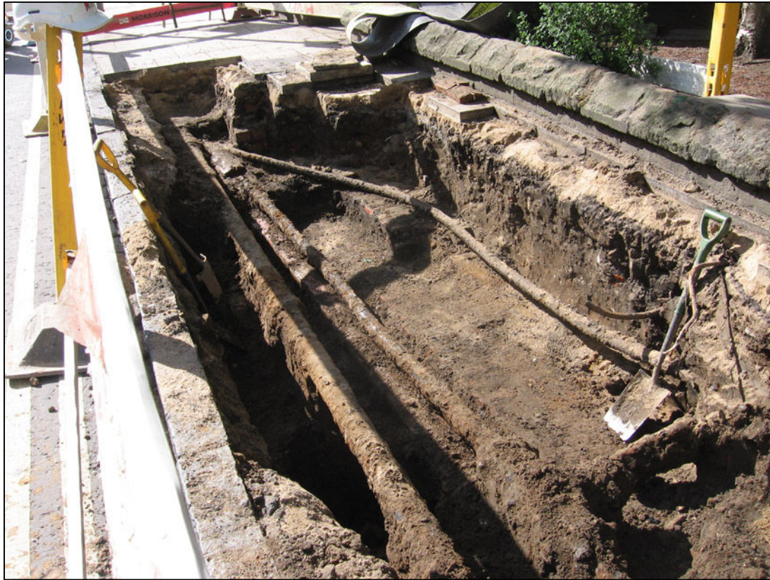
Plate 1 Trench on south-west side of Bootham, looking south-east
