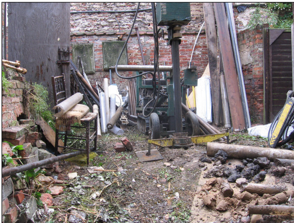
Plate 3 The borehole rig in action, looking south-east
