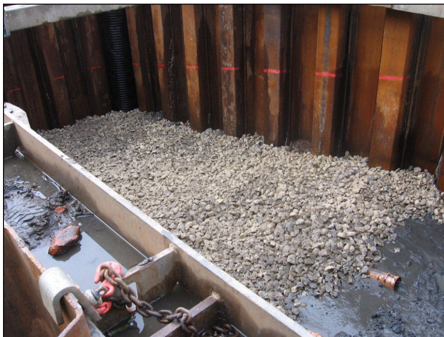
Plate 2 Stoning up within coffer dam, looking south-west
