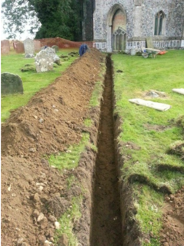
Plate 1. General view of trench, looking southeast
