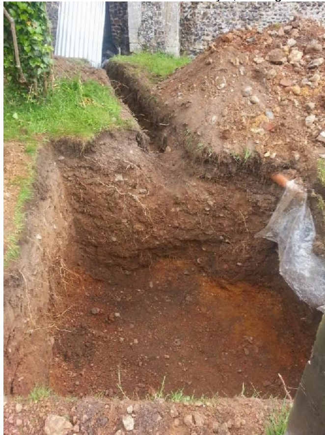
Plate 2. General view of Soakaway 2, looking north
