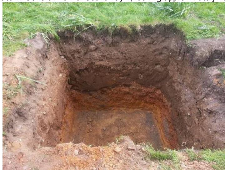
Plate 1. General view of Soakaway 1, looking approximately north
