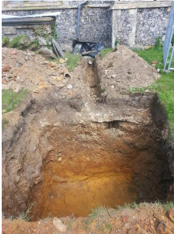
Plate 3. General view of Soakaway 3, looking north
