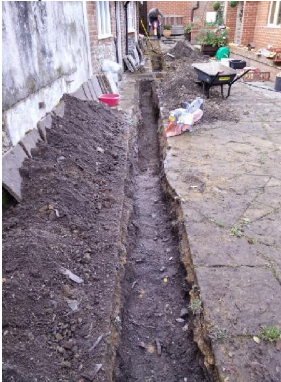
Plate 2. General view of the service trench, looking west
