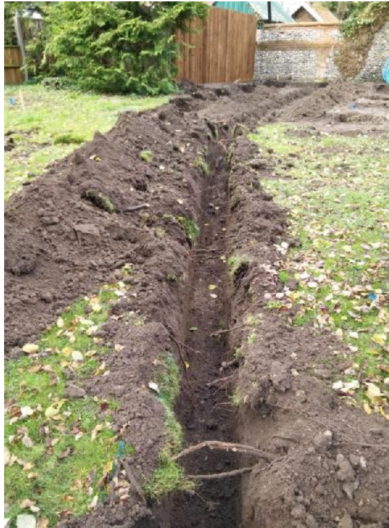
Plate 6. Excavations for the surface water drain, looking west
