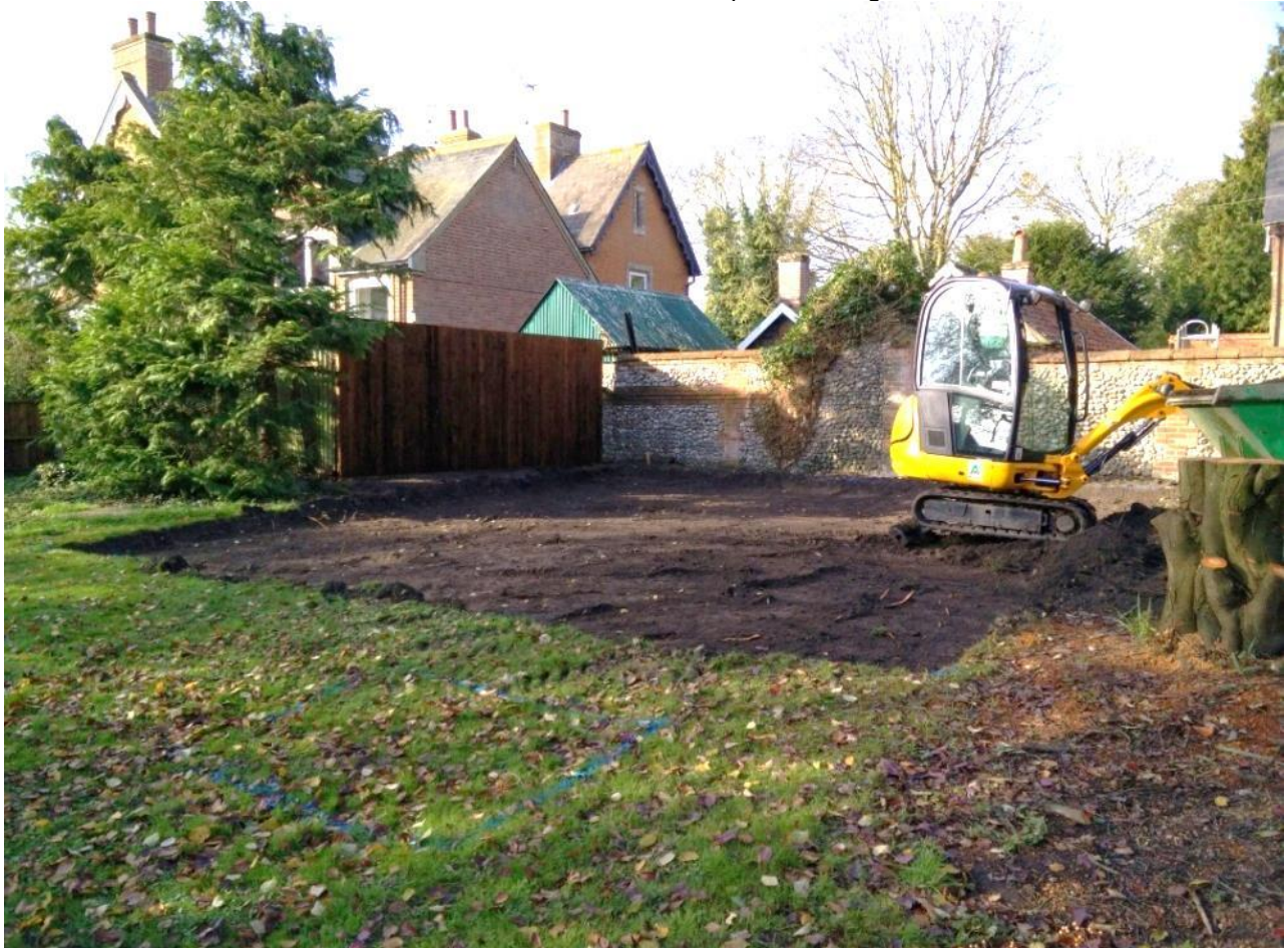
Plate 1. General view of the house footprint, looking southwest
