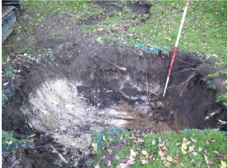
Plate 7. Excavations for the surface water soakaway, looking east
