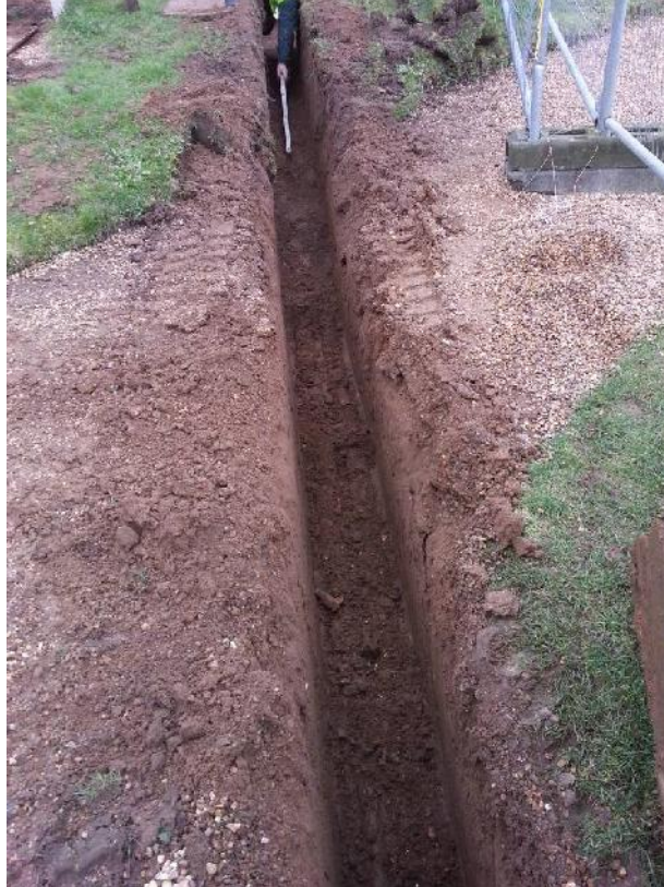
Plate 3. Sample view during excavation of the foul water trench, looking southeast
