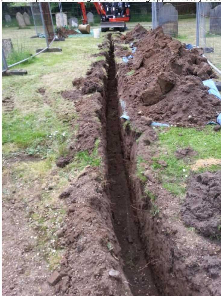
Plate 1. Example of a drainage trench, looking approximately southwest
