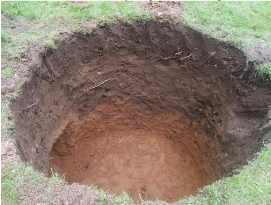
Plate 2. Example of a soakaway during excavation, looking northwest
