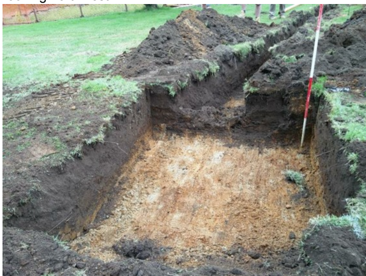
Plate 8. Example of drainage excavations, looking northwest
