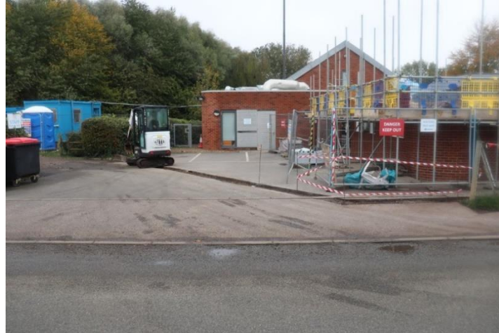
Plate 4. General view of drainage trench excavations, looking approximately northwest
