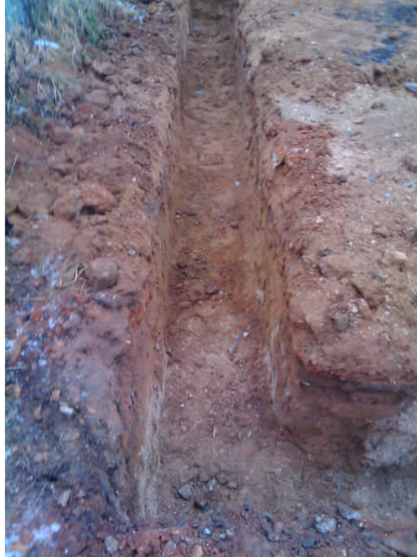
Plate 1. Example of foundation trenches during excavation, looking east
