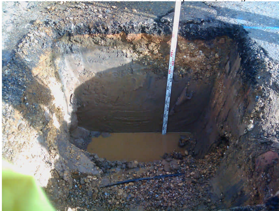
Plate 1. Excavations for foul water interceptor tank, looking north
