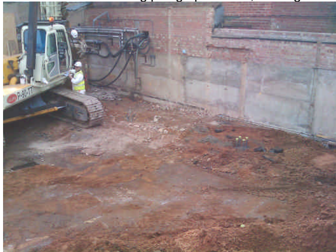
Plate 2. General view during piling operations, looking southwest
