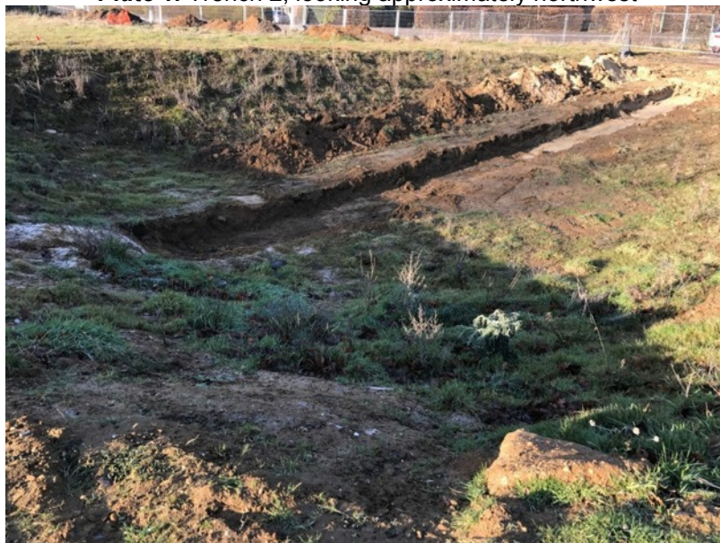
Plate 1. Trench 2, looking approximately northwest
