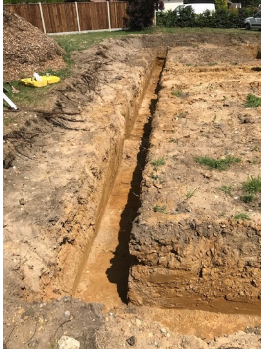
Plate 1. Example of foundation trenches, looking north
