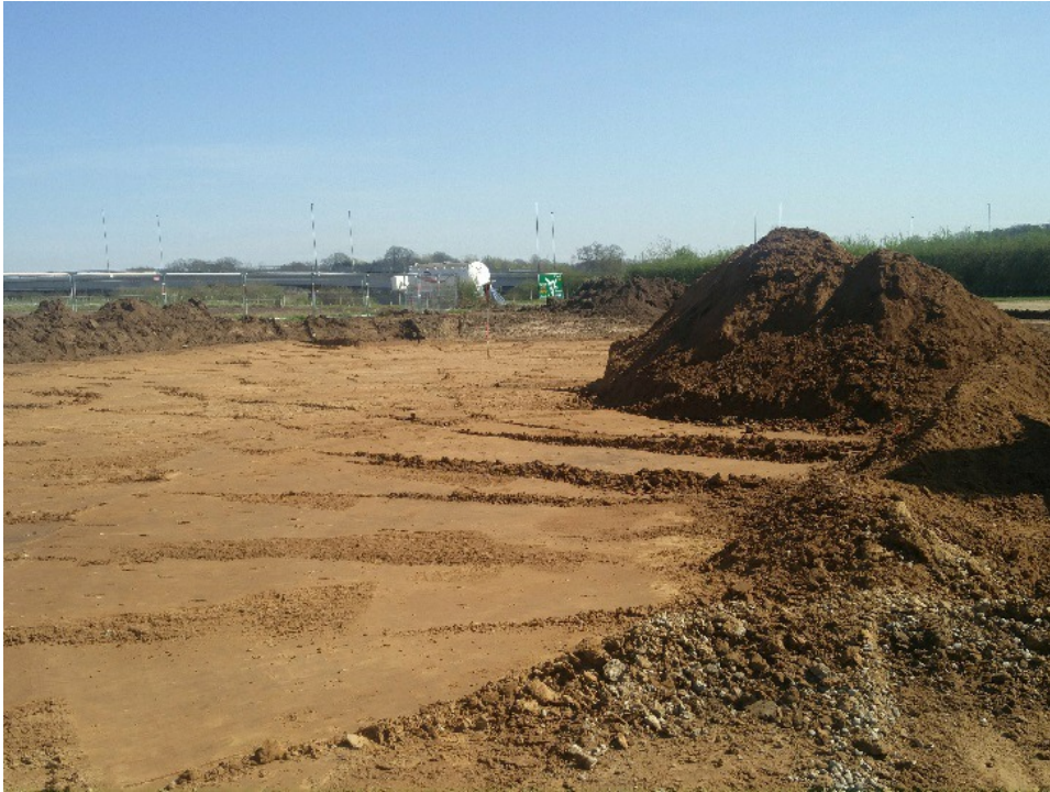
Plate 11. General view of lagoon excavations, looking southeast
