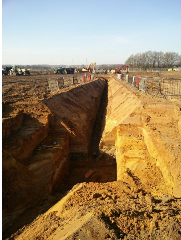
Plate 10. Sample view of drainage excavations, looking west
