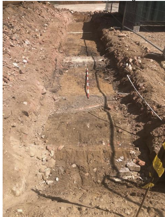
Plate 9. General view of Trench 8, looking northeast
